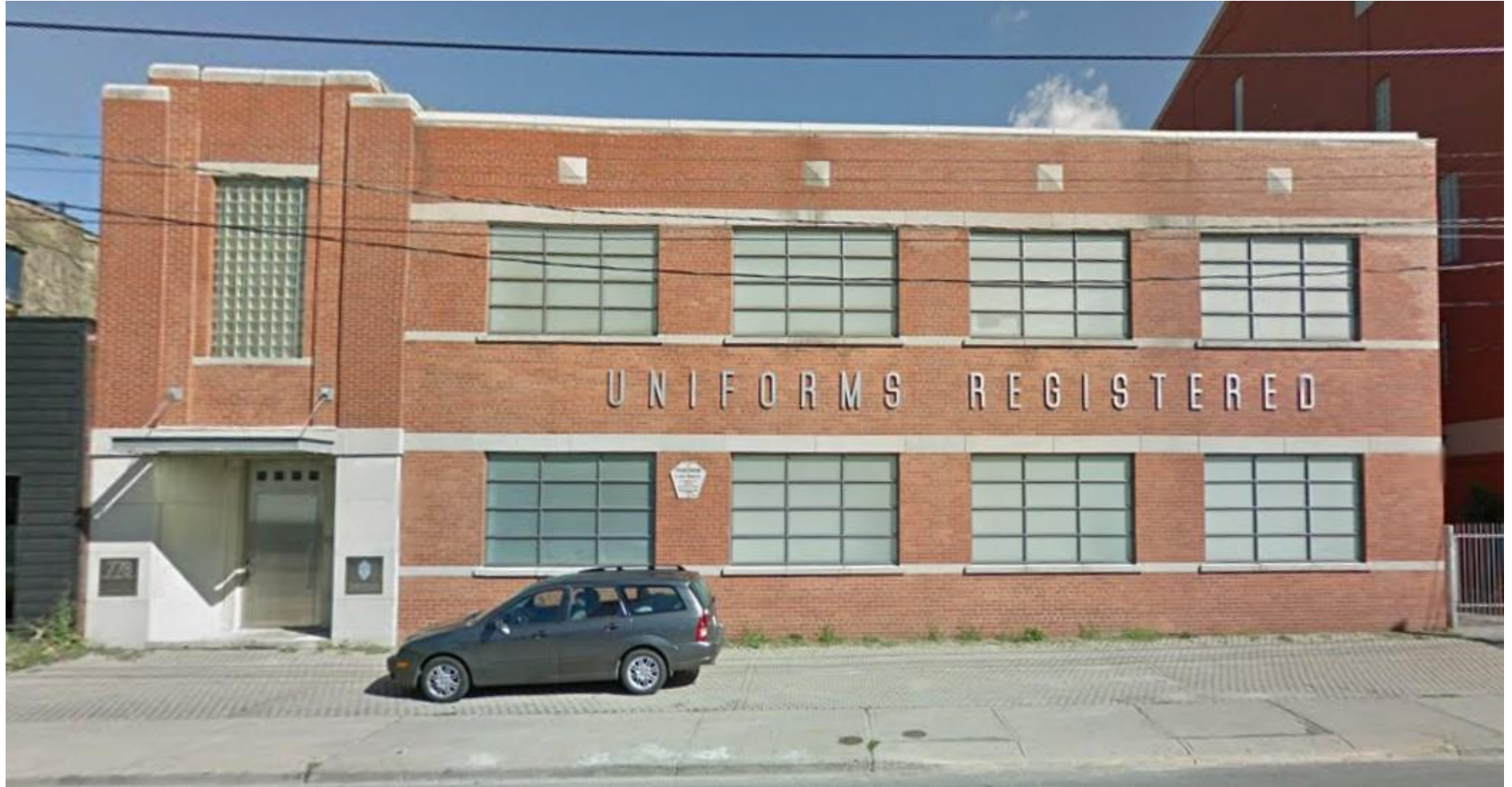
Primary elevation of the subject property, August 2011 (Google Street View).
