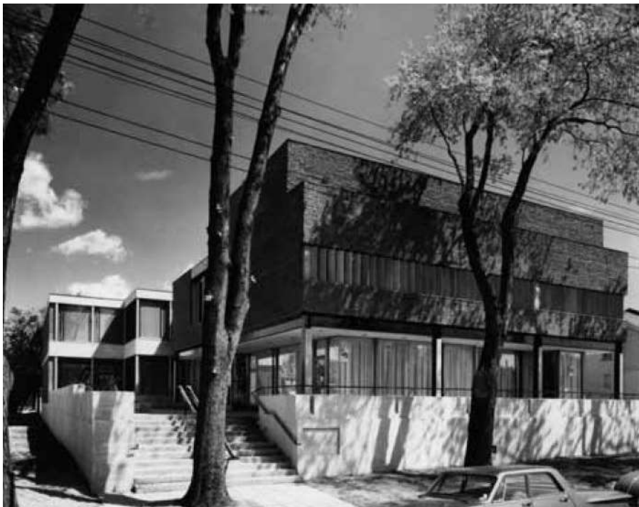
Girl Guides of Canada Headquarters shortly after completion in 1962 without the later ramp and with the original wood "brise soleil" screen on the windows at the second floor level and showing the rear office section at its original two-story height (Canadian Architectural Archives [CAA])
