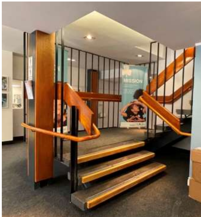
81. Main entrance lobby stair and handrail (HP, 2022)
