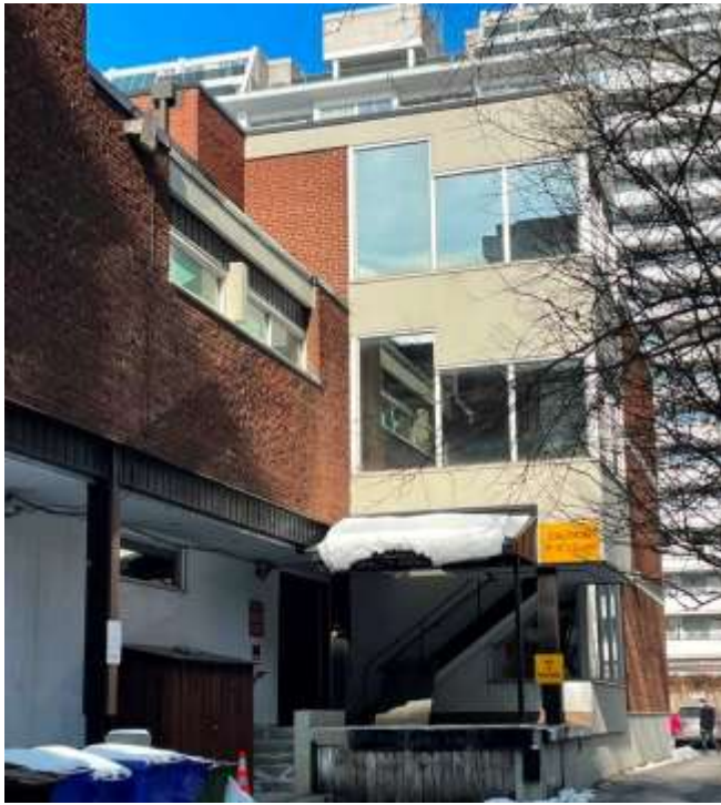
61. Fenestration on the east and south elevations showing the cut into the brick cladding to reveal the beam, the windows and the concrete fin and beyond, curtain wall glazing of the office section applied to the 1970 fire escape staircase. (HP, 2022)
