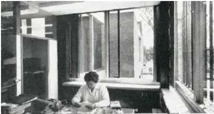
92. Corner office, second floor looking south and showing original opening sections and glass and plywood partitions and the integrated shelving above the HVAC system ( Canadian Architect , September 1962, p 48)
