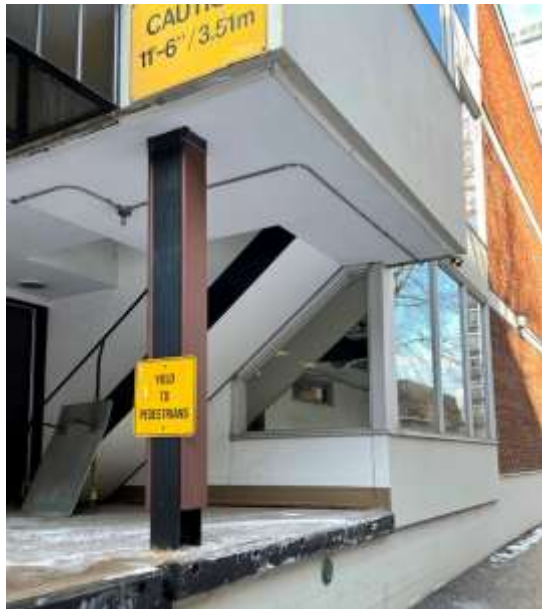
63. Steel column with wood cladding on the loading dock (HP, 2022)
