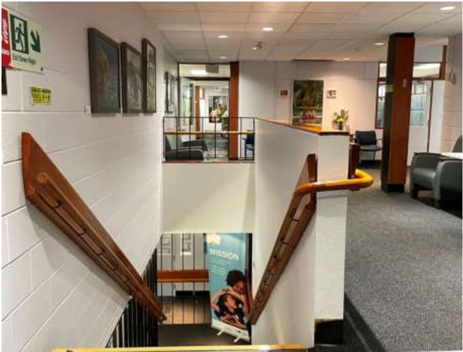
83. Staircase, handrails and balustrade at the second floor level (HP, 2022)
