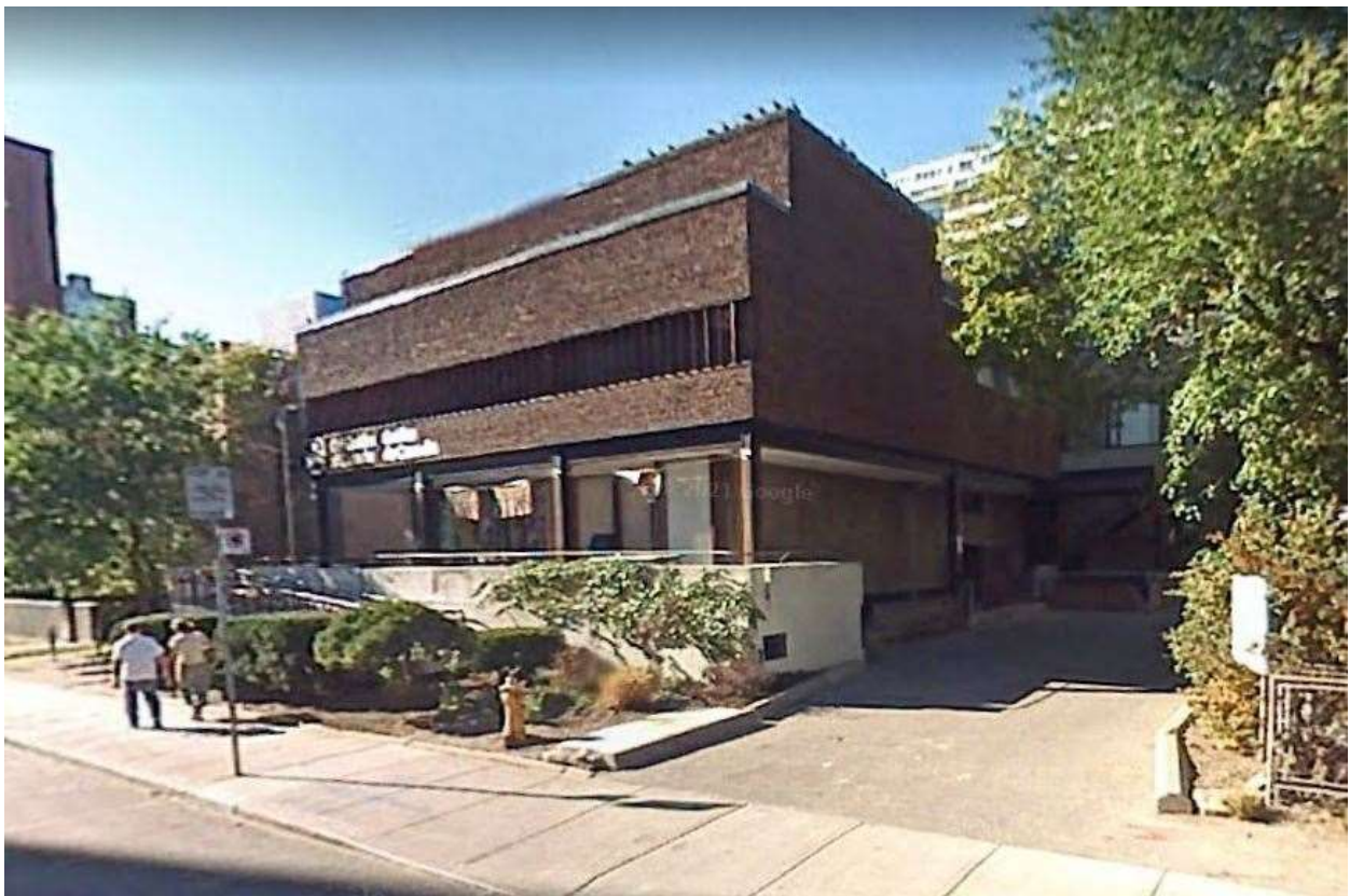
66. South and east elevations of the Girl Guides' headquarters, with the ribbon windows of the piano nobile , recessed first floor behind a screen of columns, here in an urban location with a raised podium, brick cladding and, a screen of wood fins (Google Street View, 2007)
