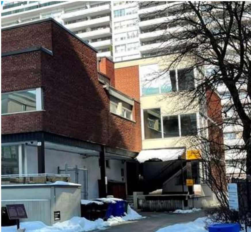
68. Principal, south and side, east elevations showing loading dock and driveway access (HP, 2022)
