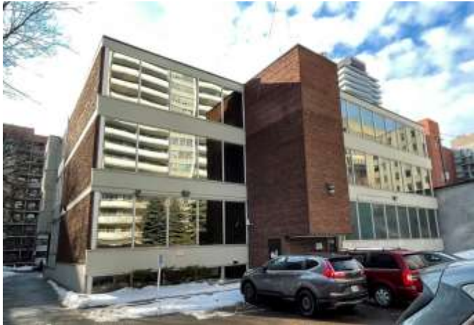
71. North and east elevations showing the rear, north side with the projecting, brick-clad volume of the staircase and third floor addition completed in 1970 (HP, 2022)
