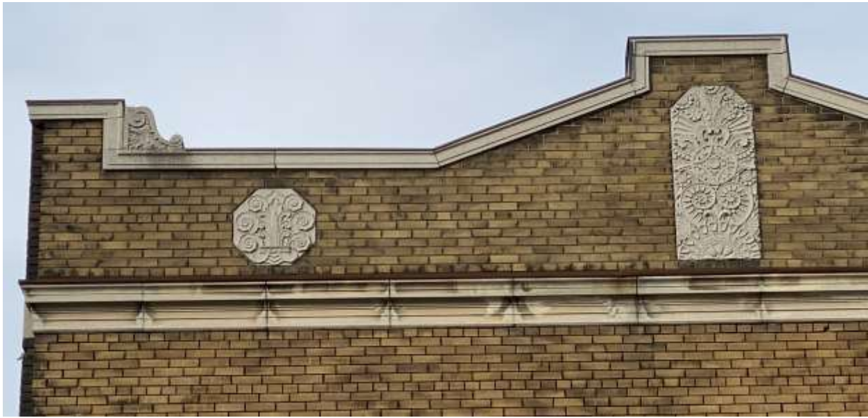
Image 16. Detail view of southernmost section of segmented parapet roofline with stone capping above and stone banding below. Stone corbel and two stone spandrel panels with floral motif visible. (Heritage Planning, March 2022).
