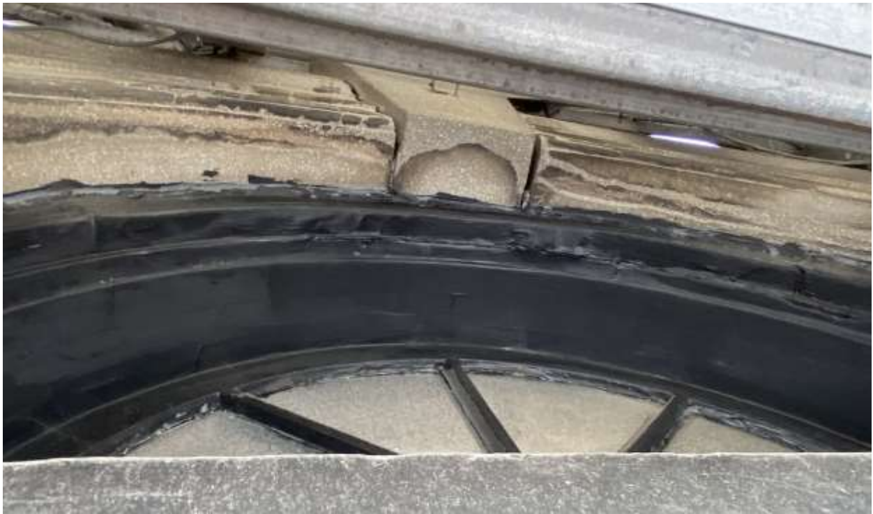
Image 14. Detail view of arched, fan-light transom window above the southernmost side entrance at 1420 Yonge Street. (Heritage Planning, March 2022).
