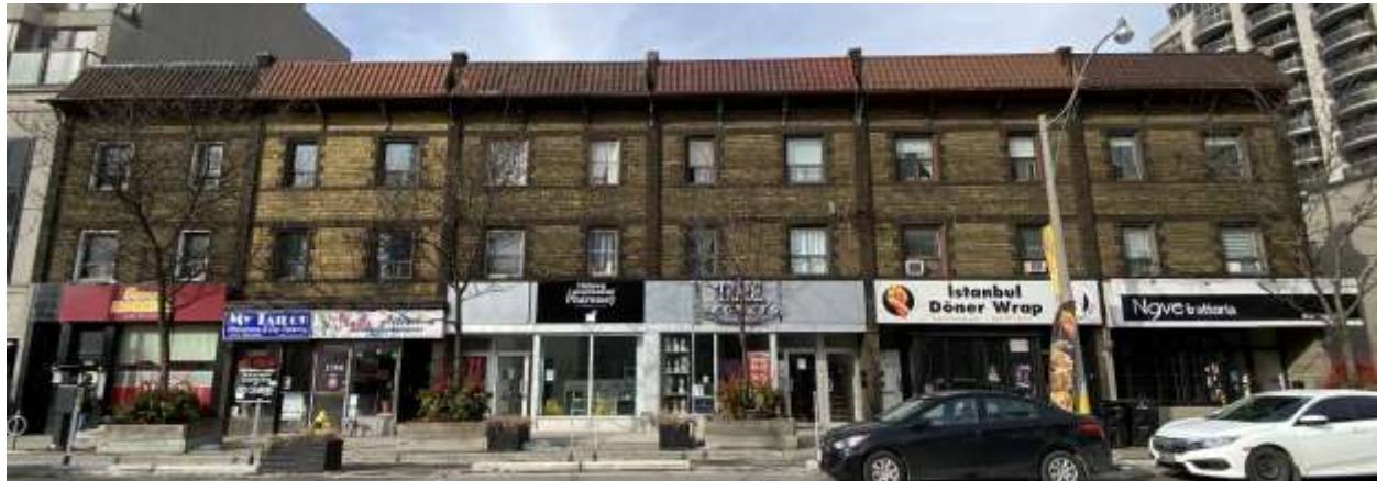
East (principal) elevation of the main street commercial row at 1390-1406 Yonge Street (Heritage Planning, March 2022)
