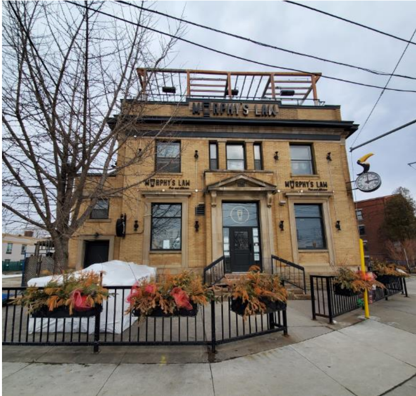
1702 Queen Street East located at the northwest corner of Queen Street East and Kingston Road
