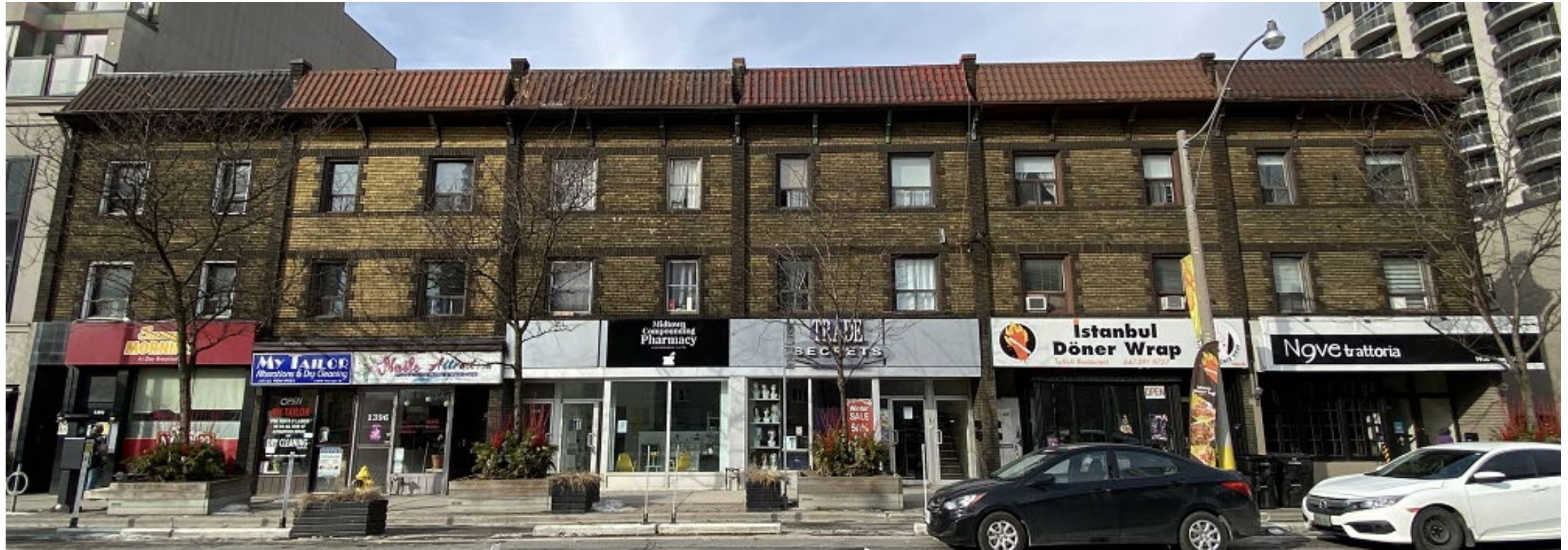
Principal (east) elevation of 1390-1406 Yonge Street (Heritage Planning, 2022)
