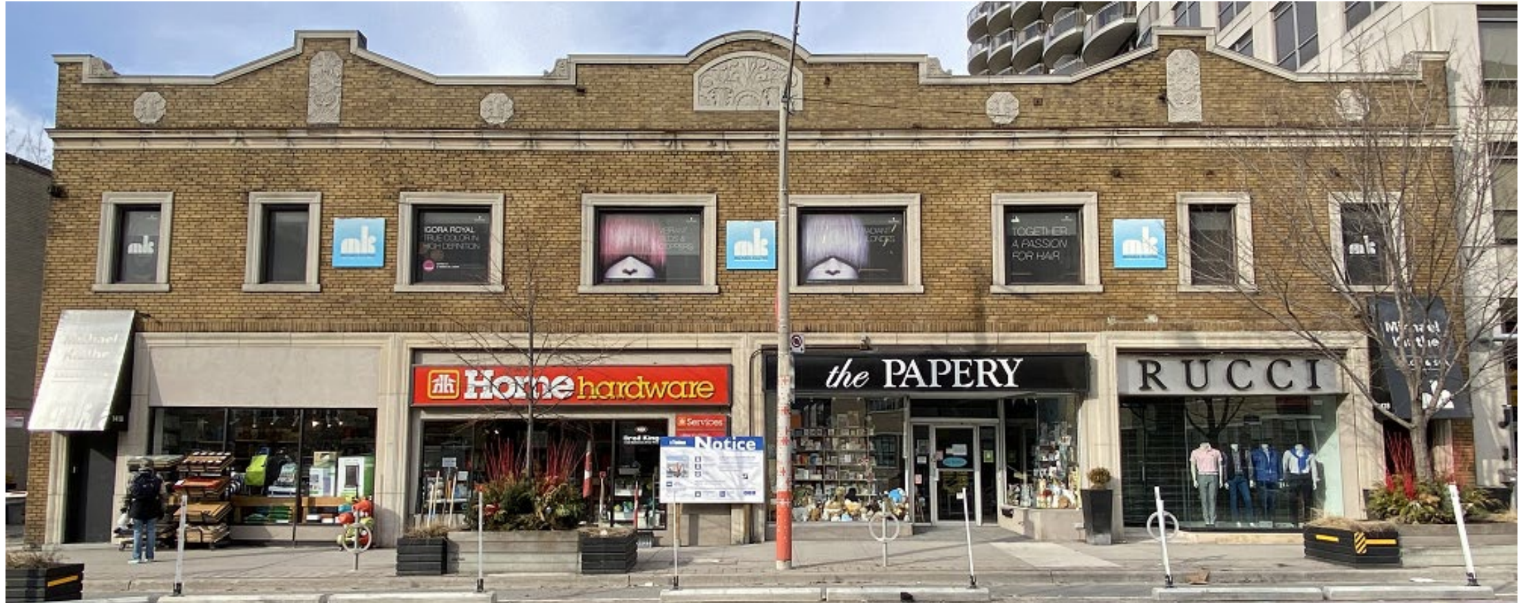
Principal (east) elevation of 1420 Yonge Street (Heritage Planning, 2022)
