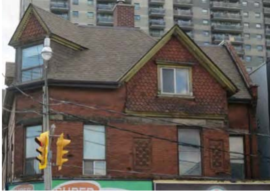
21 and 22. Details at 148 Avenue Road: the asymmetrical roofline, brick cladding, rough stone banding, decorative terracotta fish-scale shingling in the gables and inset terracotta panels at the upper levels (left); detail of one of two decorative glass transoms flanking the main entrance (right). (ERA)
