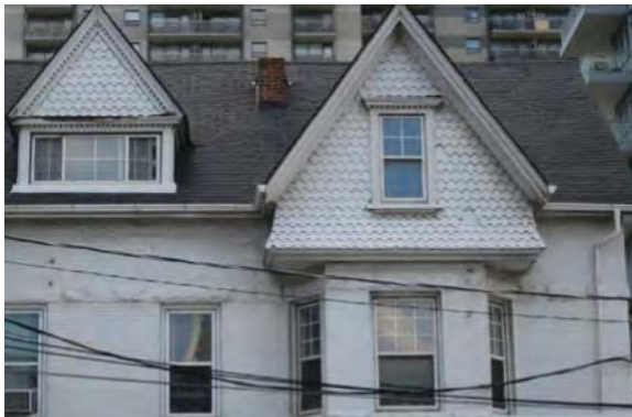
23 and 24. Details at 156-158 Avenue Road: the brick cladding, rough stone banding, and bay window (left); decorative wooden window frame detailing with dentils and terracotta fish-scale pattern shingling in the gables (right). (ERA)
