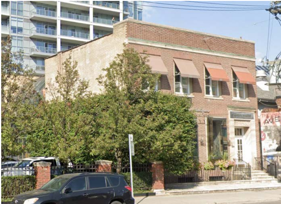
26. Current image of the Canada Bread Building at 224 Davenport Road showing the stone and copper cornice line on the principal (south) elevation and buff brick cladding on the west elevation. (Heritage Planning, 2021)
