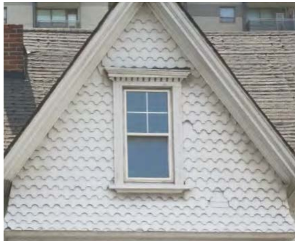
23 and 24. Details at 156-158 Avenue Road: the brick cladding, rough stone banding, and bay window (left); decorative wooden window frame detailing with dentils and terracotta fish-scale pattern shingling in the gables (right). (ERA)
