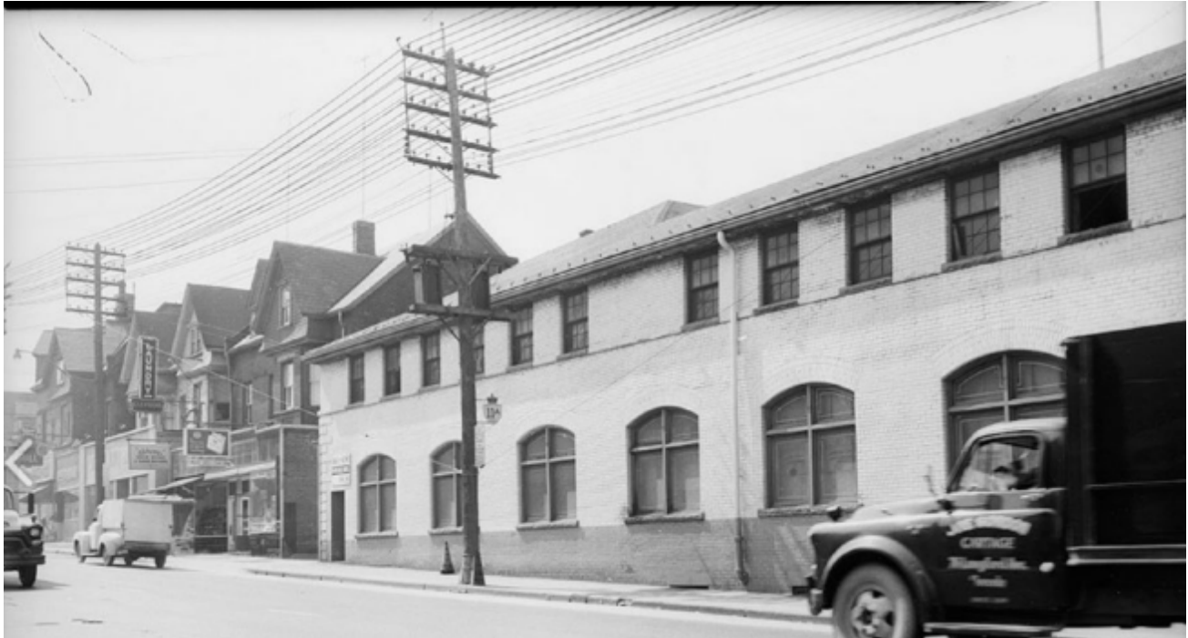
13. 1959 archival photo from the Avenue widening showing the properties at 148-158 Avenue Road at left and the Bredin Bread Company bakery in the foreground at 160-164 Avenue Road (demolished). (CTA)
