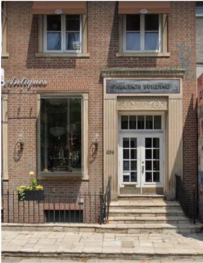
25. 224 Davenport Road: detail of raised main entrance on the principal (south) elevation showing the stone door surround with fluting pilaster and carved inset, decorative window surrounds and metal railing. (Heritage Planning, 2021)
