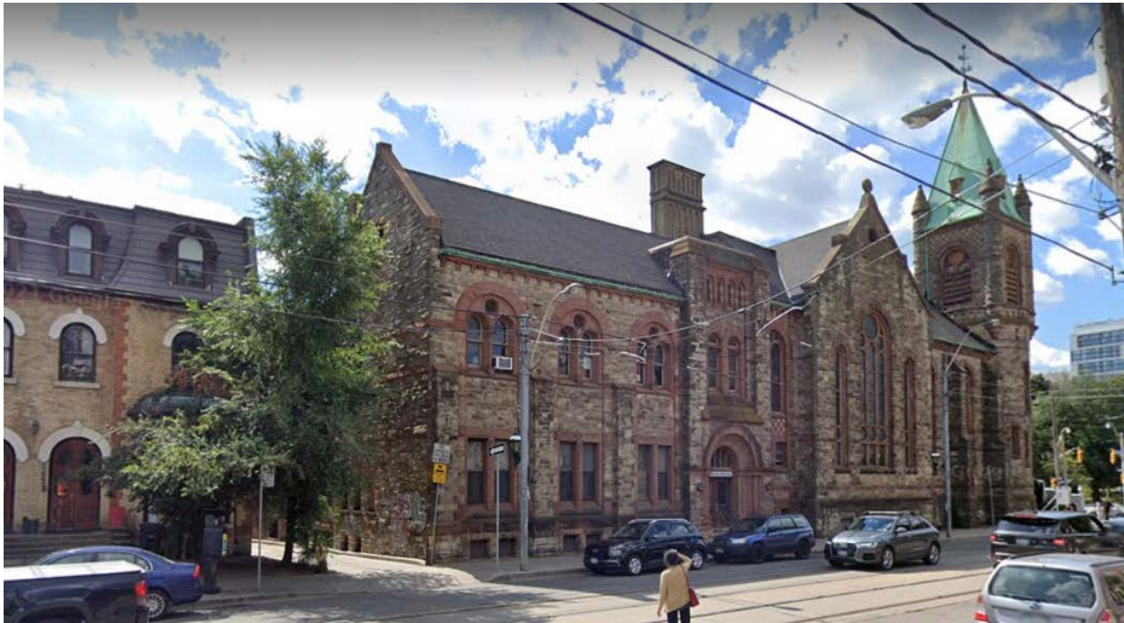
View of the north (Carlton Street) elevation
