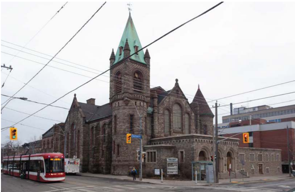
View of the north and west elevations
