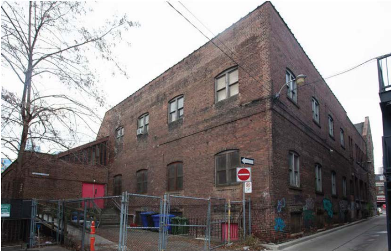
View of the east and south elevations of the Sunday school (Source: ERA Architects)
