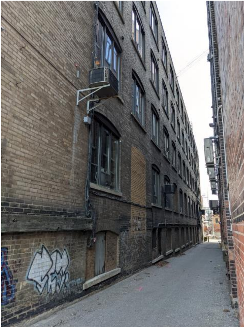
Figure 13. Partial view of the side (west) elevation looking south (Heritage Planning, 2022)
