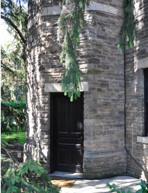
Tower at the southeast corner, exterior (ERA 2017).
