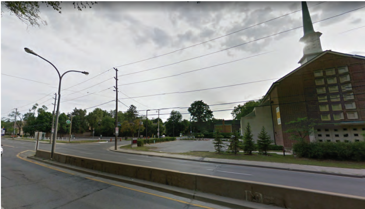
Southwest-facing view across Bayview Avenue, with the Lawrence Park Community Church in the foreground, and the north edge of the large townhouse development at the left edge of the frame (Google Streetview, 2016).
