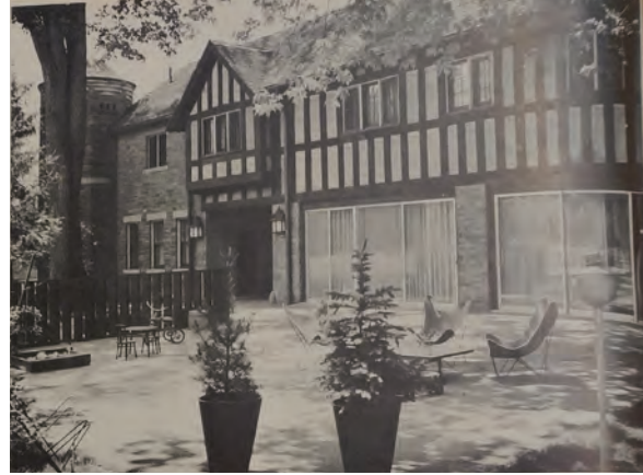
East elevation prior to the carriageway's enclosure (Ontario Homes and Living, 1963).
