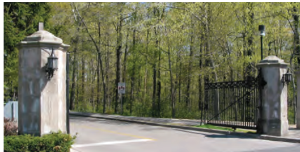
Gates to the Wood estate - Glendon Hall (ACO Toronto, 2016).
