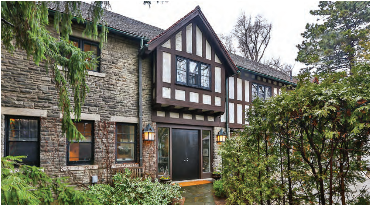
East elevation, view from northeast (Amantea Architects 2017).
