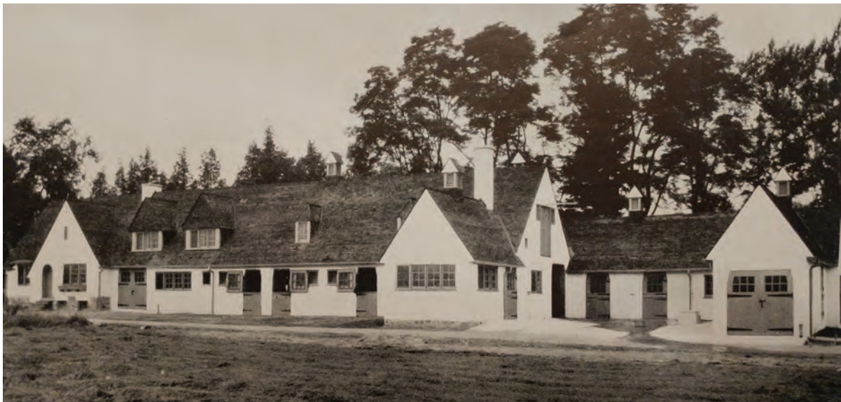
South elevation of the stables and garage, south of the estate driveway, designed by Wickson & Gregg, 1929 ( Canadian Homes & Gardens , May 1929).
