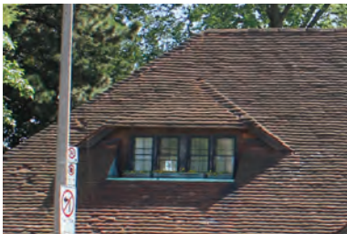
Dormer window, 2nd storey (ERA 2017).
