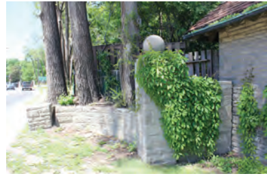
Stone wall, north portion (ERA 2017).
