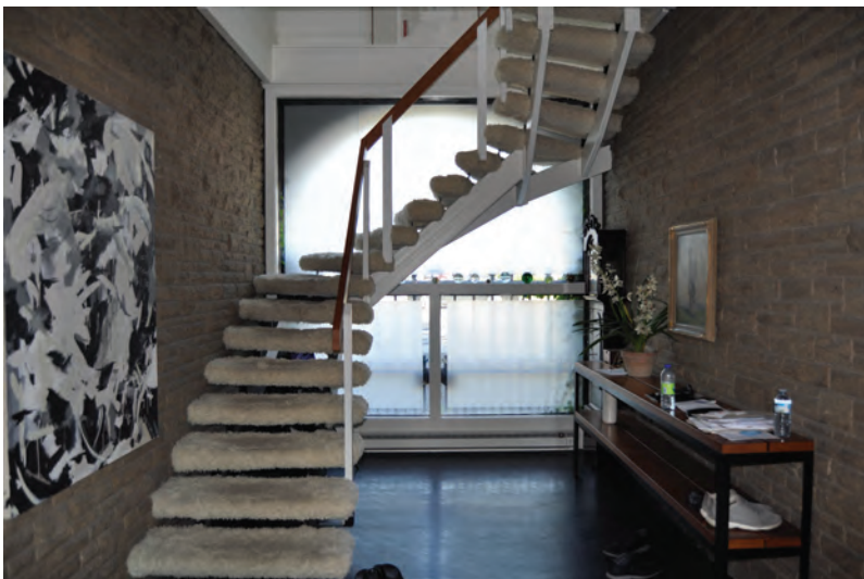
Inside the currently-enclosed carriage-way, facing west. The semi-transparent glazing within the archway added in the mid 1960s (ERA 2017).
