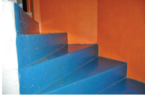
Winding staircase inside the tower(ERA 2017).
