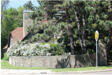
Stone wall, south portion (ERA 2017).
