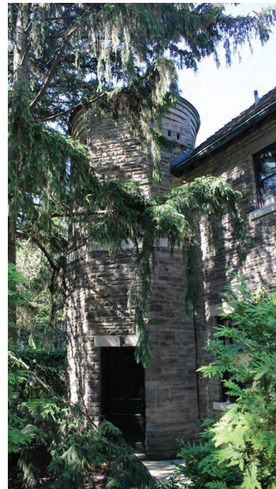
Tower, view from northeast (ERA 2017).
