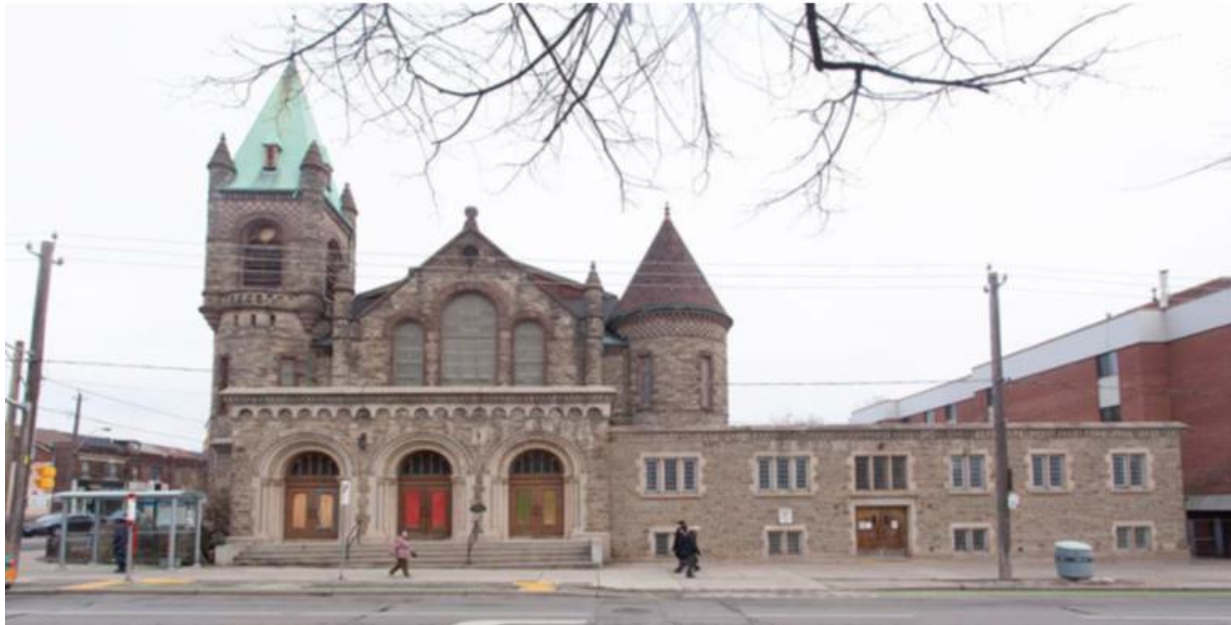
West (Sherbourne Street) elevation
