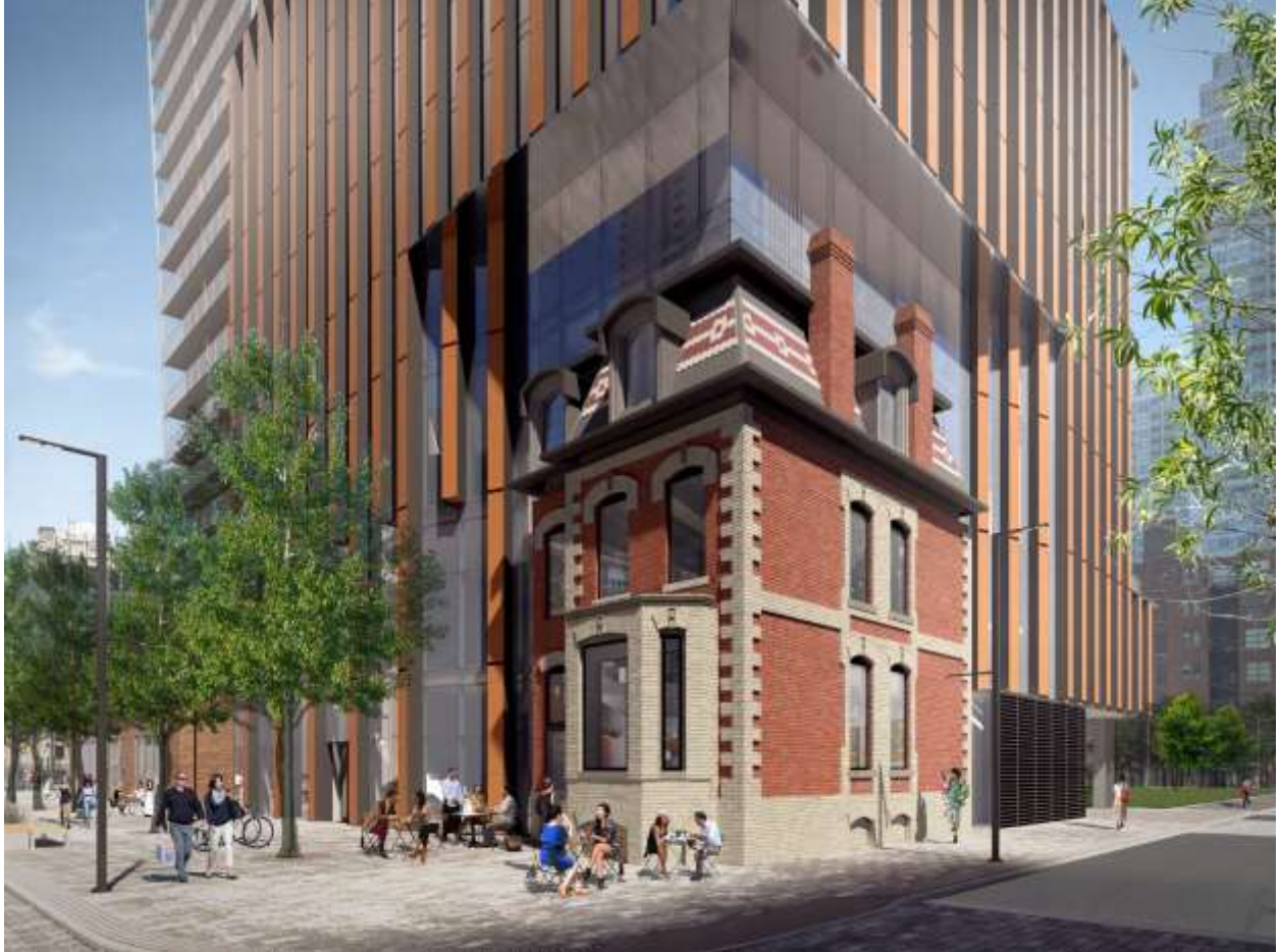
Render showing 133 John Street. Missing heritage features will be reintroduced. Window types will utilize profiles appropriate for age and style of the property.
