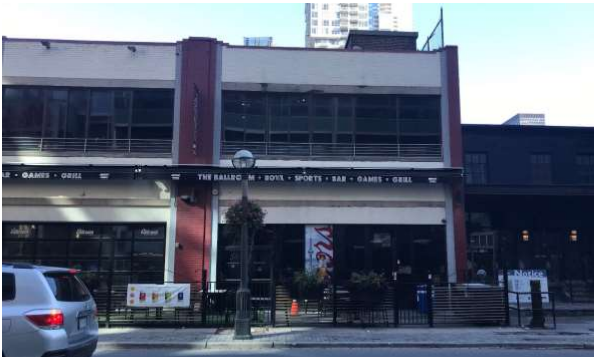
Current photograph showing the additional bay constructed in 1948 at the southern end of the west elevation. This bay will be removed.
