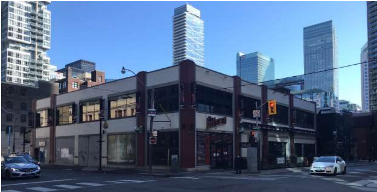
Current photograph of the building at 241 Richmond Street West from the northwest and showing the principal (west and north) elevations.
