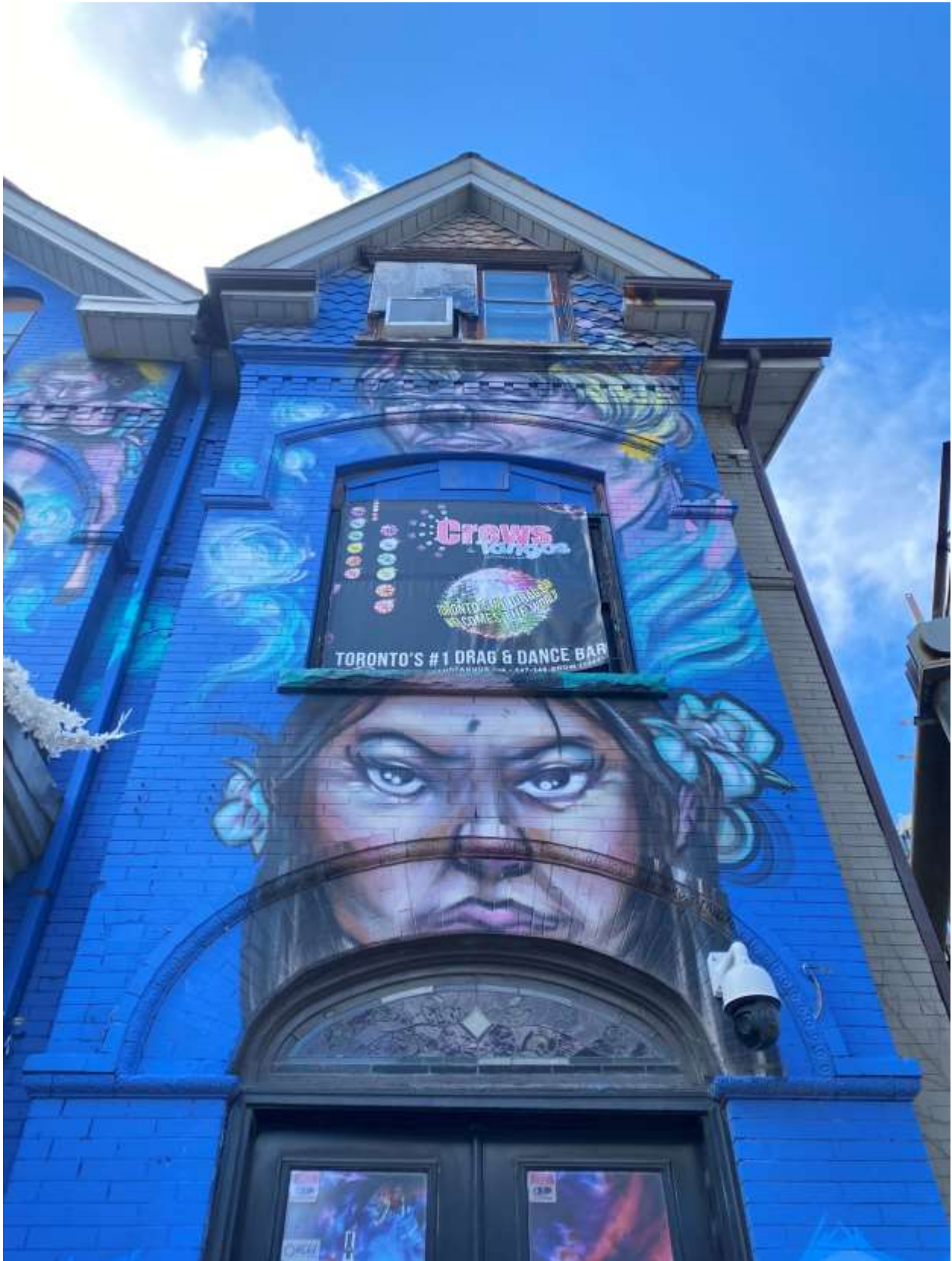
Architectural detailing on the northernmost bay of the front elevation, 2022 (Heritage Planning).
