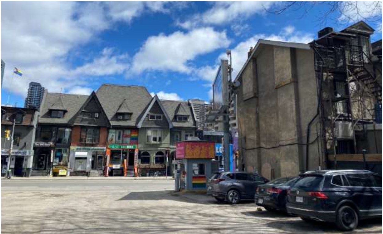
Eastward view from the parking lot immediately north of the subject property, with its north and rear elevations visible at right, 2022 (Heritage Planning).
