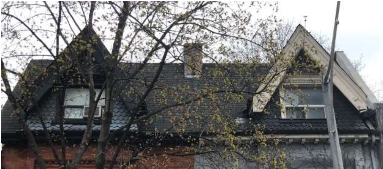
Image 12. Current photograph showing the second- and attic- storeys of the subject properties. The shared roofline, attic storey form, arrangement, style and materials at the subject properties are all original. (Heritage Planning, 2021)
