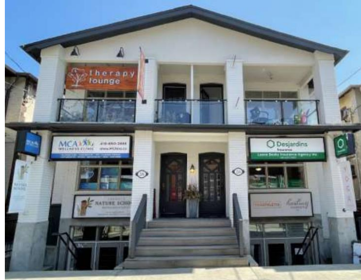
2243 Queen Street East
