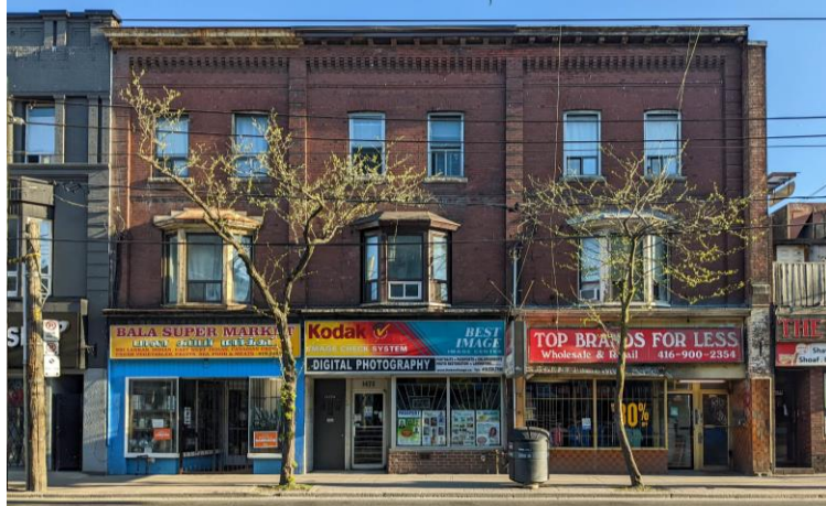
1468A-1474 Queen Street West, 2022
