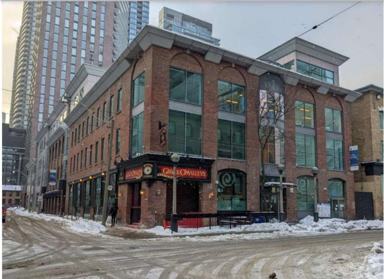
View of the southeast corner (Heritage Planning, 2022)
