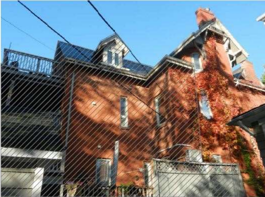
Partial view of east elevation showing the area at rear proposed for demolition
