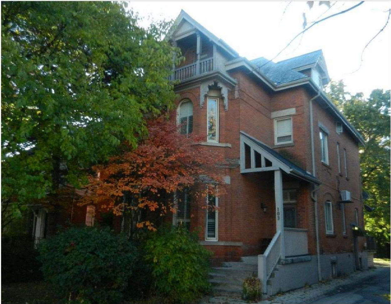
Partial view of the north (principle) elevation of 103 Heath Street
