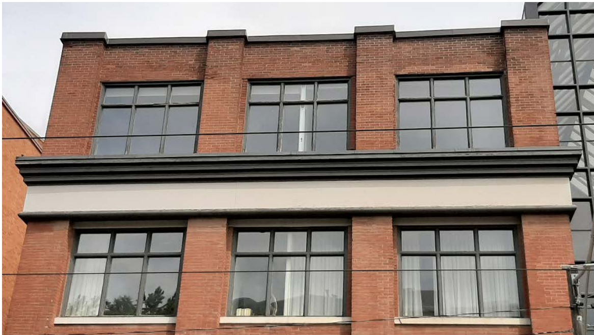
Image 18. Cornice detail upon the former National Electric Heating building (today part of 544 and 550 Queen Street East). Heritage Planning, 2022.
