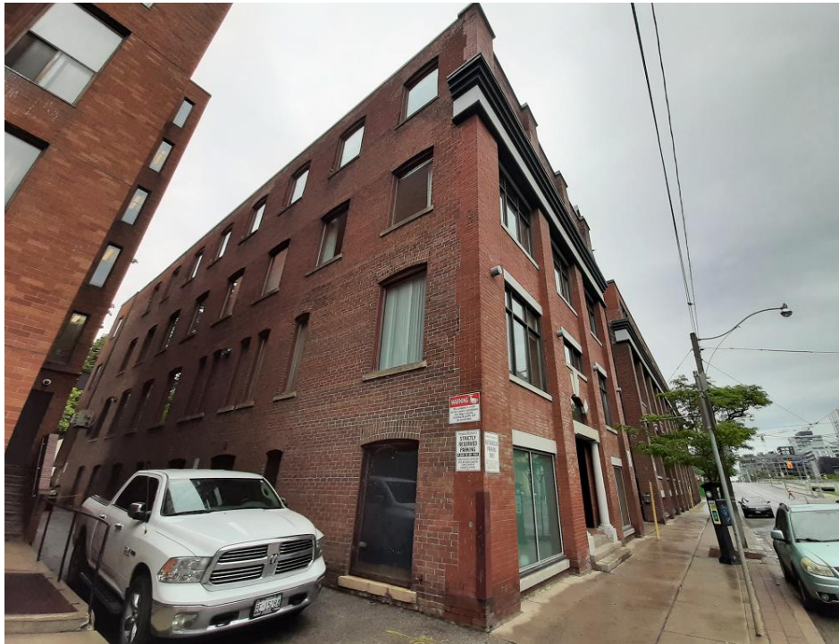
West elevation of the former National Electric Heating building (today part of 544 and 550 Queen Street East). Heritage Planning, 2022
