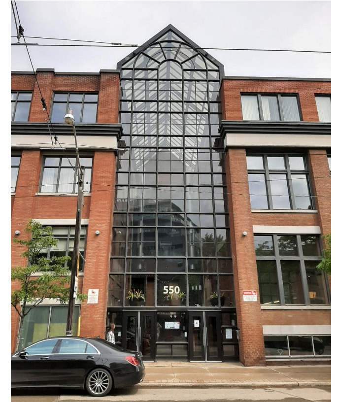
Atrium connecting the former National Electric Heating and New Method Laundry buildings which comprise 544 and 550 Queen Street East. Heritage Planning, 2022.
