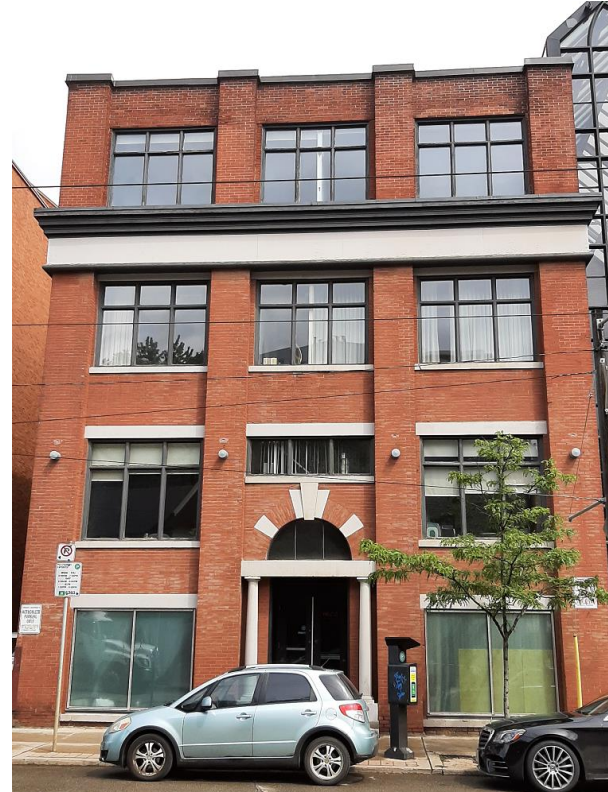
Front elevation of the former National Electric Heating building (today part of 544 and 550 Queen Street East). Heritage Planning, 2022.
