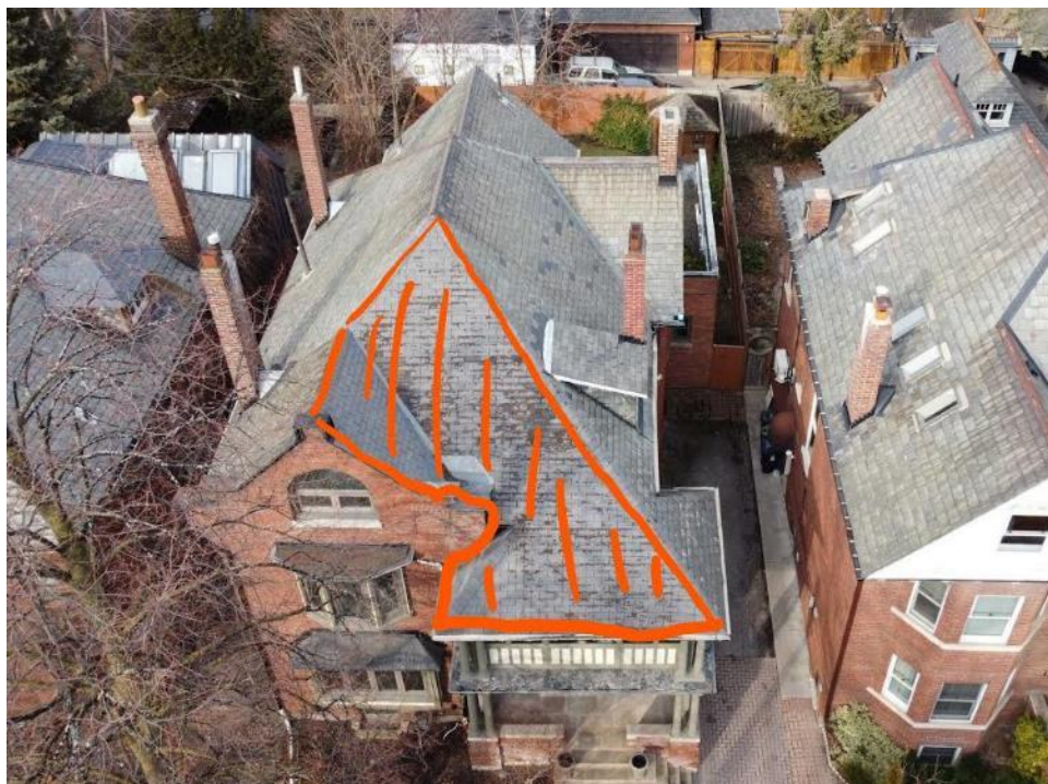
Slate Roof replacement and restoration
