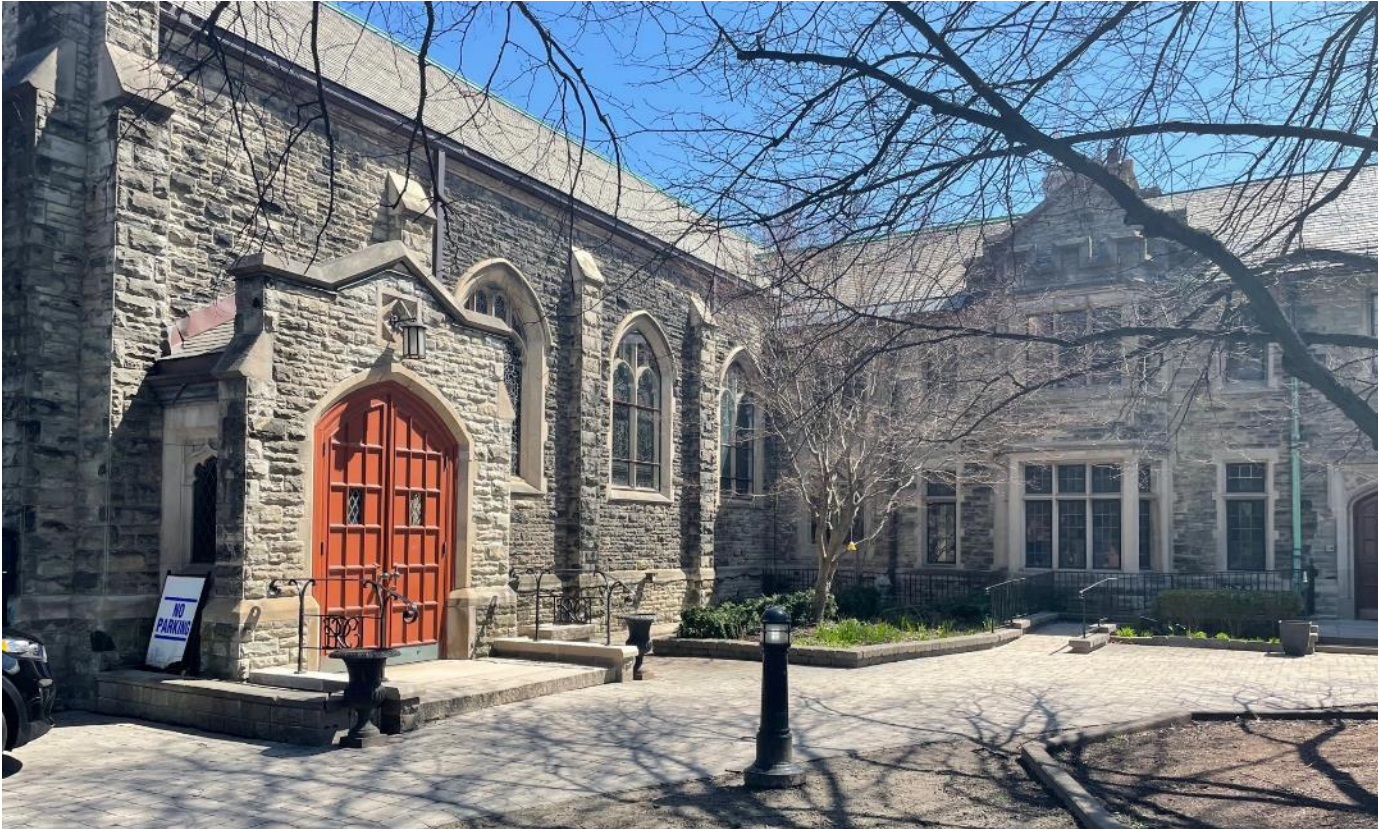
Restoration of stained glass windows
