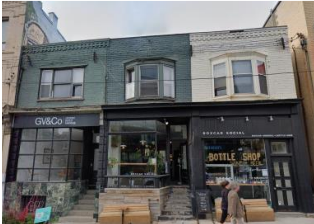
2021 Image showing the east elevations of the commercial main street row at 1206-1210 with their bay windows and decorative brick detailing in the upper storey and post-1914 raised entry stairs (external at 1206-1208 and internal at 1210).
