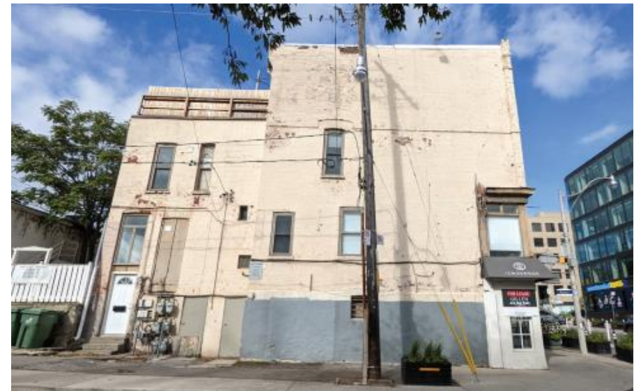
2021 Image of the south elevation of the corner property at 1196 Yonge (including 2 Birch Avenue) and showing the alterations to openings in the 1920s and a floating doorway at left that serves as a reminder of the earlier street grade.
