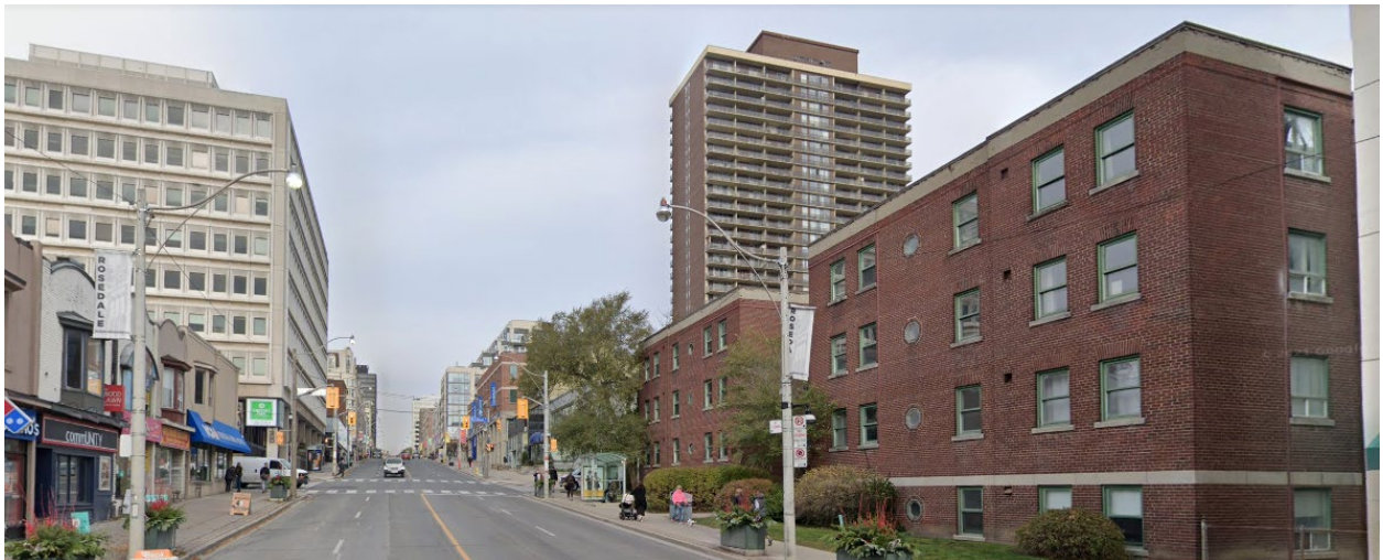
Yonge Street looking north to the intersection of Woodlawn Avenue. 1223 Yonge (on the right, east side of the street) (Source: Google Streetview 2020)
