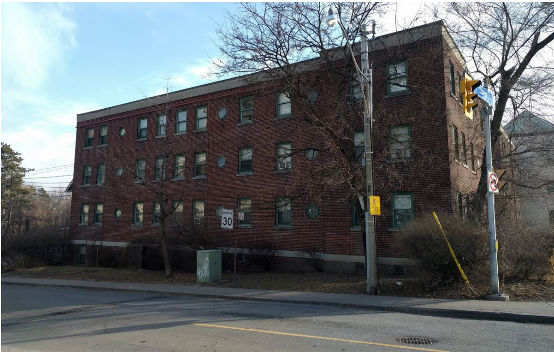
North elevation of 1233 Yonge Street taken from Woodlawn Avenue East (Source: ERA Architects).
