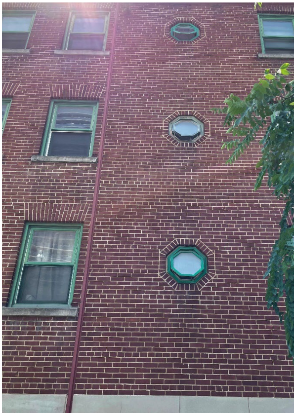
Octagonal windows (Heritage Planning July 2022)
