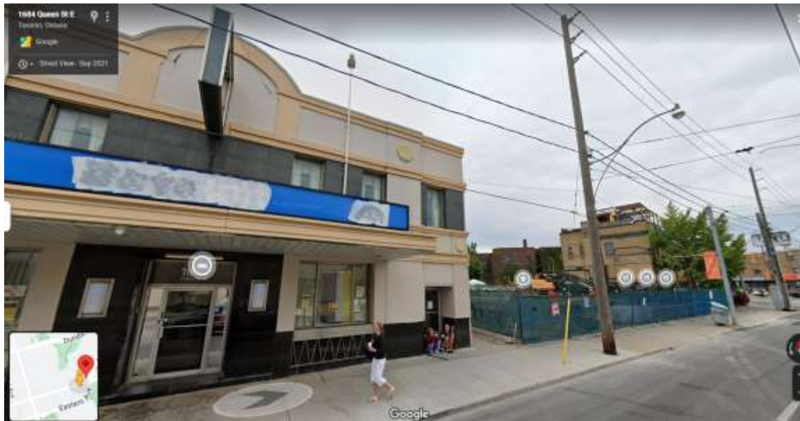
Looking north east into existing site - Google Street View (September 2021)
