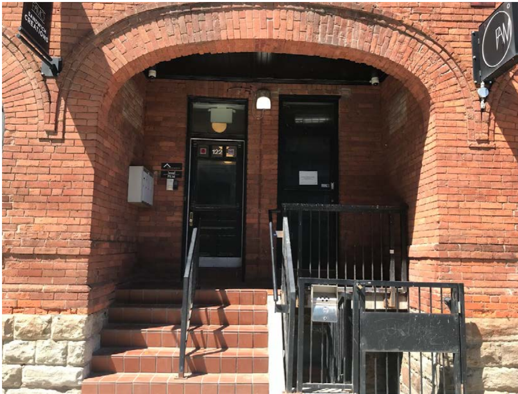
Image 19. Current photo showing the main entry to the properties at 120-122 Sherbourne Street, with their shared, centre arch brick entryway containing two raised and recessed doorways. (Heritage Planning, 2022)
