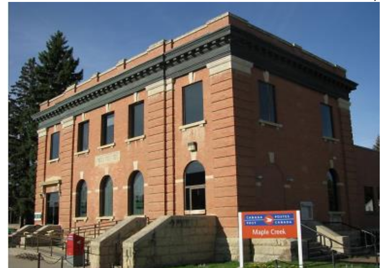
Post office, Maple Creek, Saskatchewan (Town of Maple Creek website)
