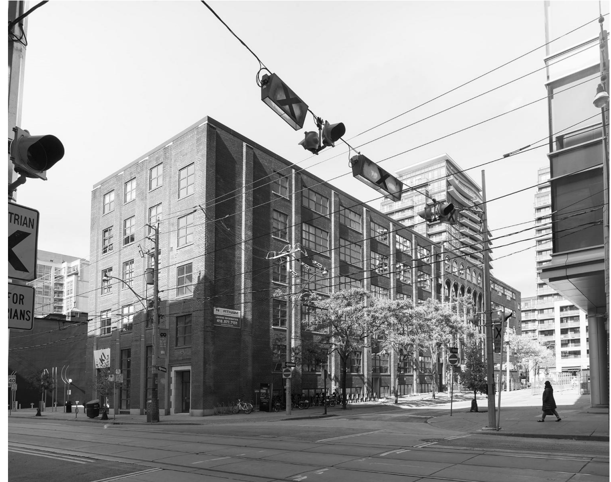
266 King St E (Source: City of Toronto, 2020)
