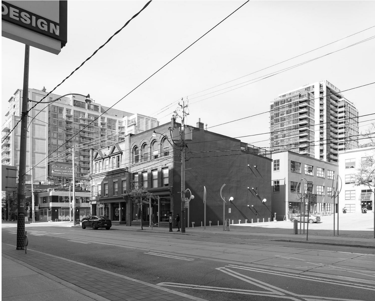
254 King St E & 256 King St E (Source: City of Toronto, 2020)
