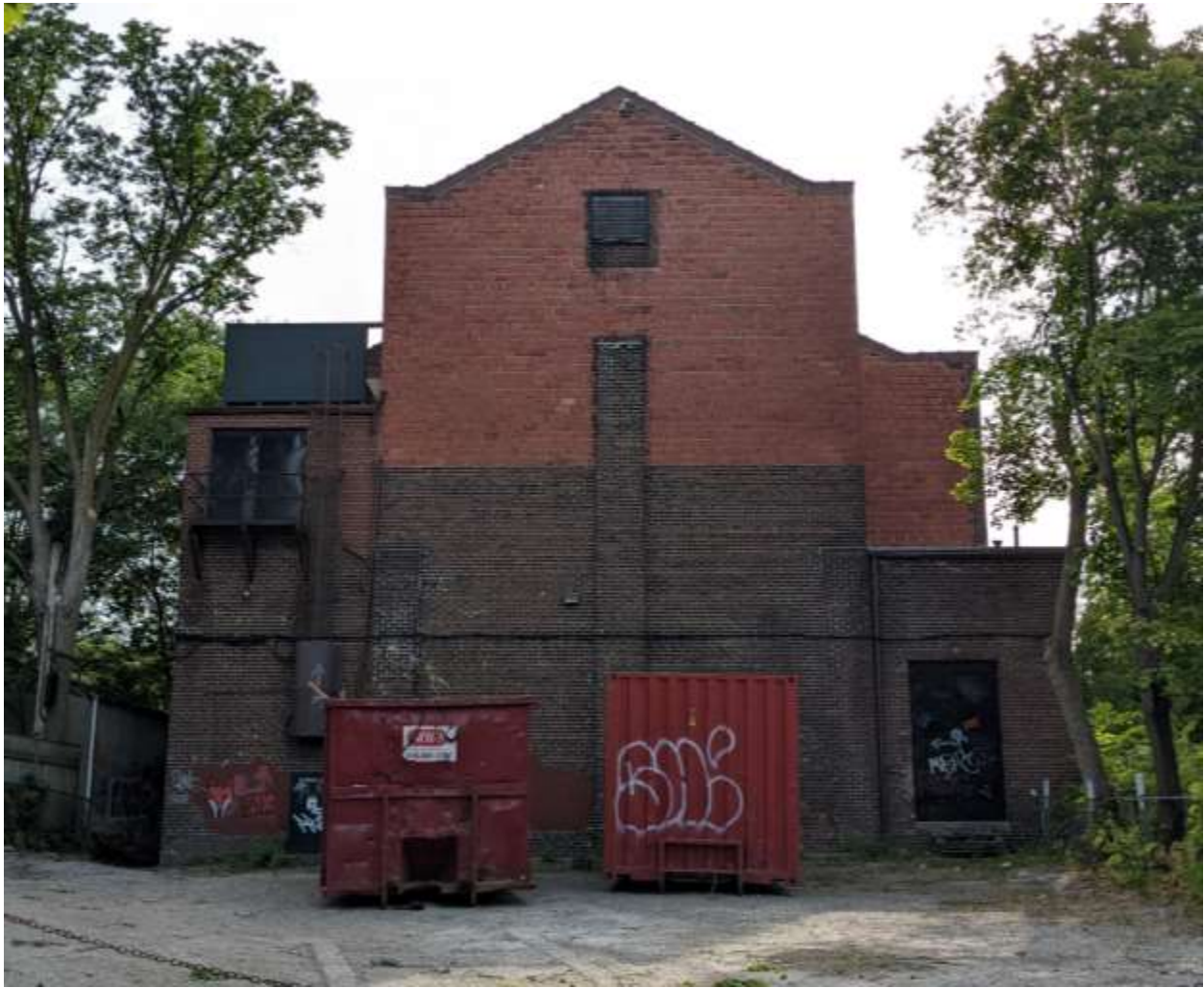
Figure 16. Rear (east) elevation of 551 Mount Pleasant (Heritage Planning, 2022).
