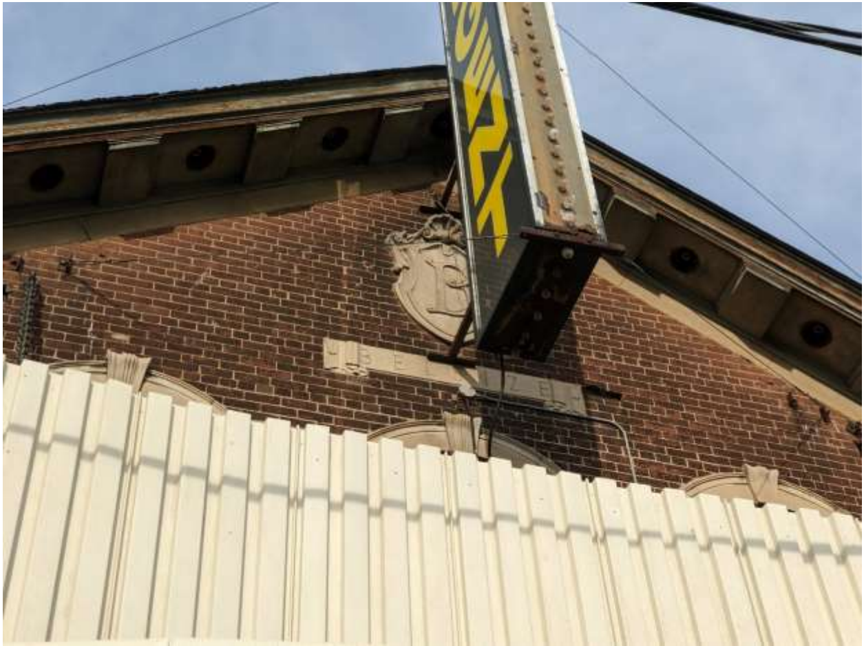
Figure 18. Detail of the front elevation, showing the carved stone crest and inscription (Heritage Planning, 2022).
