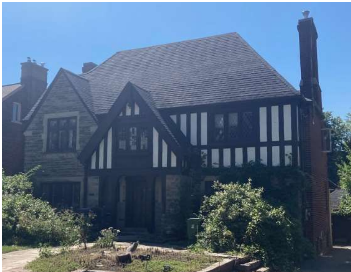
Image 4. 14 Rosemary Lane. Front (north) and side (west) elevations. Heritage Planning, 2022.
