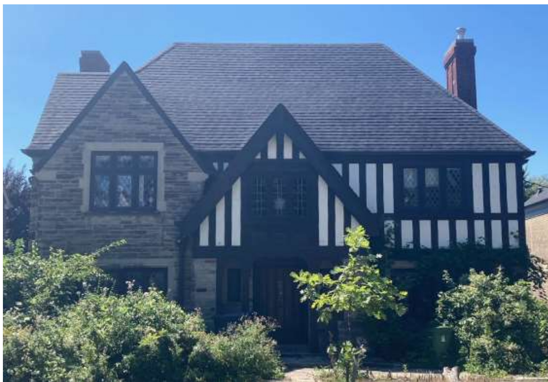
Image 3. 14 Rosemary Lane. Front (north) elevation. Heritage Planning, 2022.
