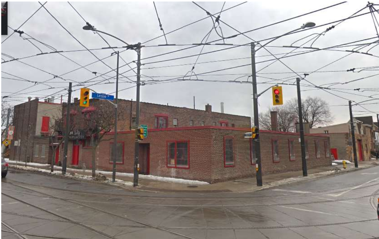
Figure 36: View of the subject property from February 2018. (Google Street View)
