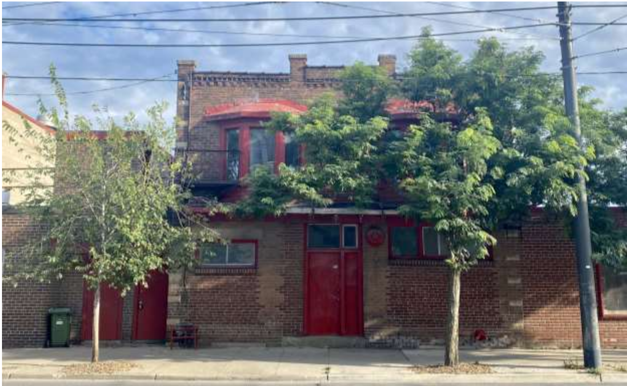
Figure 29: North elevation of the 1920-1921 structure, with the 1950 addition visible at left, 2022. (Heritage Planning)
