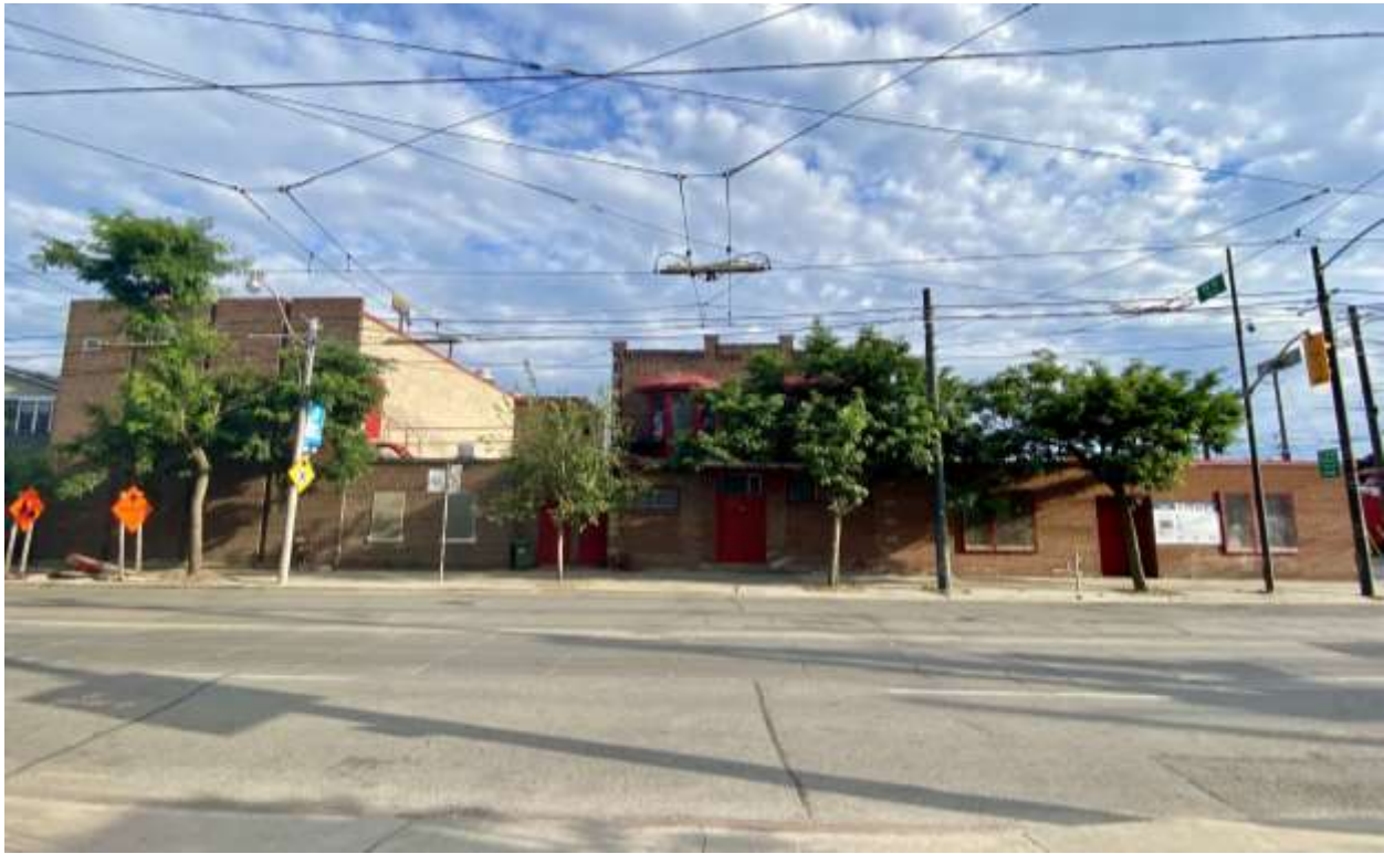
Figure 31: North elevation of 1233-1235 Queen Street East along Leslie Street, 2022. (Heritage Planning)
