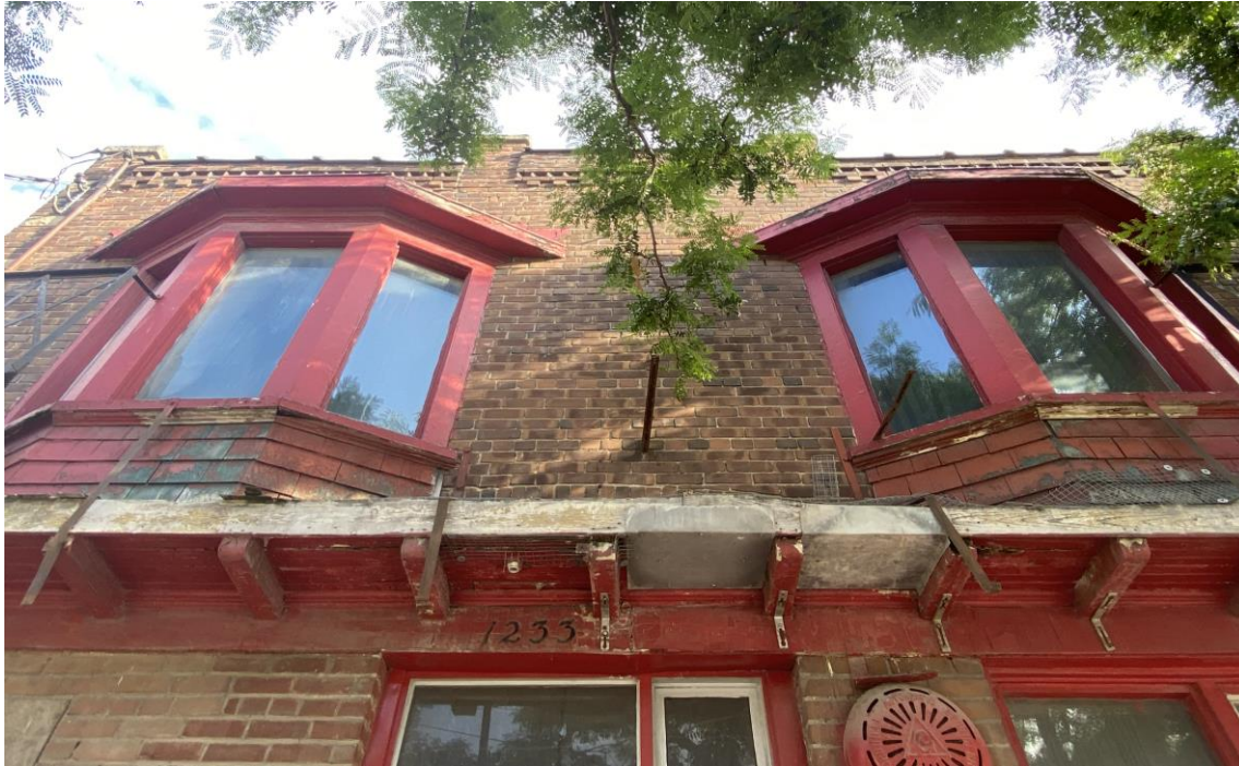
Details of the 1920-1921 structure, 2022. (Heritage Planning)
