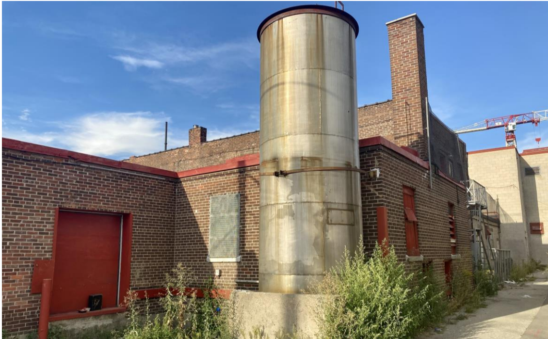
Southwest corner of the subject property, showing the c.1956 addition and 1960 steel tank, with the oldest (1920-1921) structure visible beyond, 2022. (Heritage Planning)
