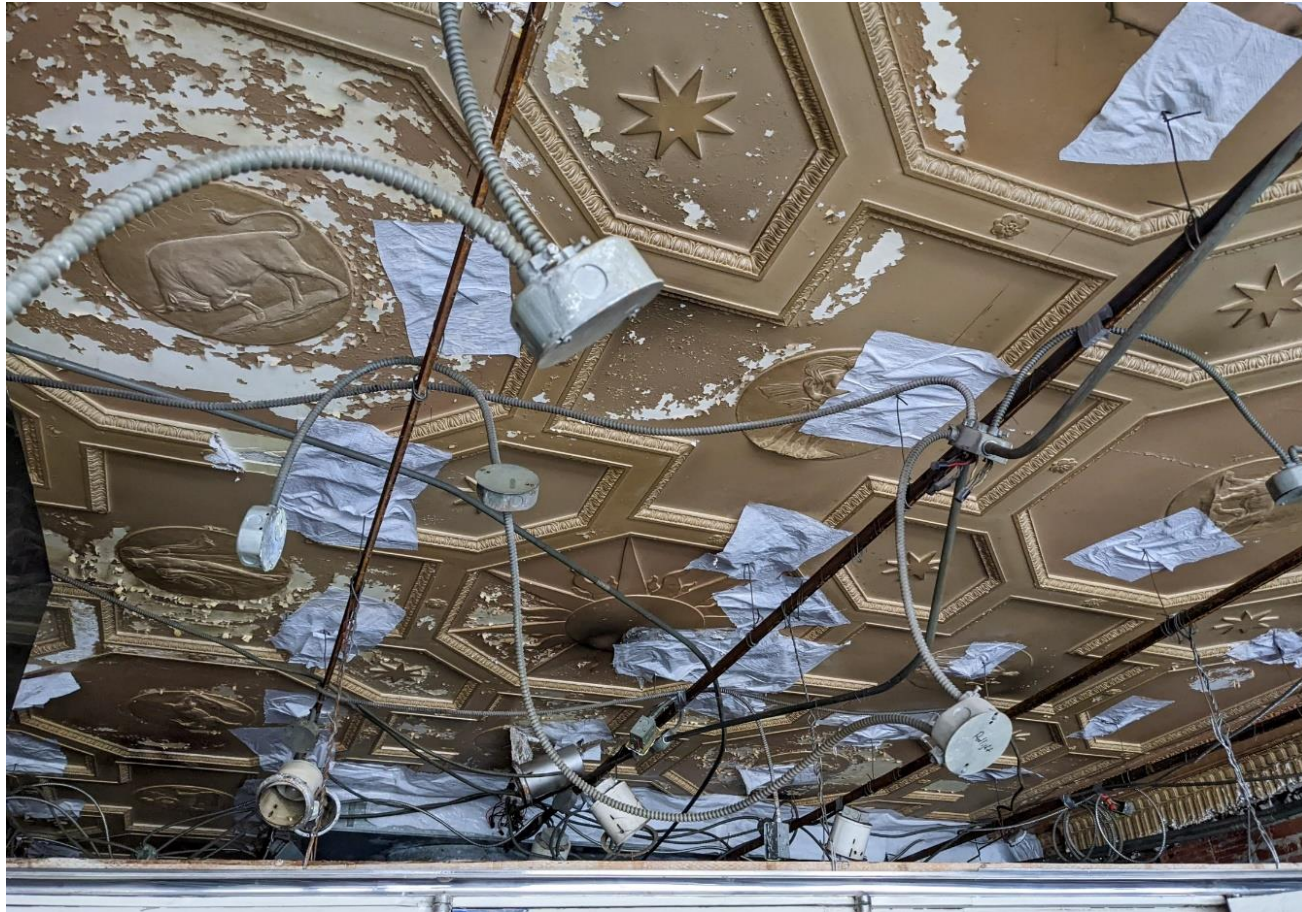
Partial lobby ceiling previously concealed (Heritage Planning, 2022)
