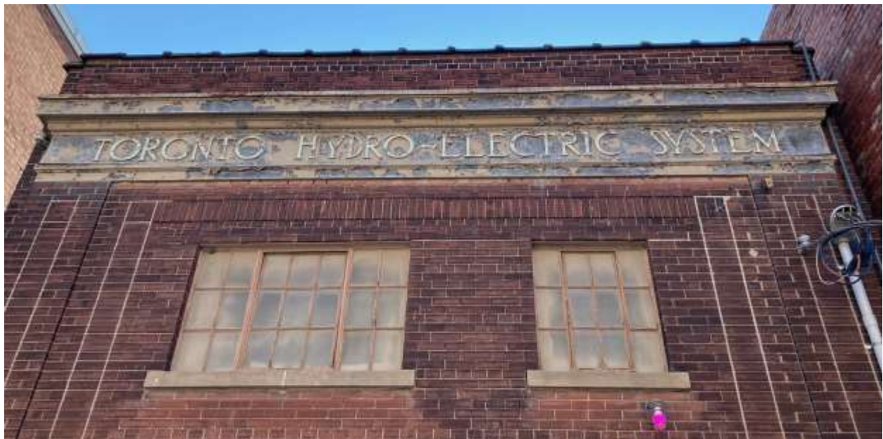
Image 12. Close-up view of 18 Portland Street. Note the metal entablature with sign band, factory type windows, brick masonry details, and terracotta coping. Heritage Planning, 2022.
