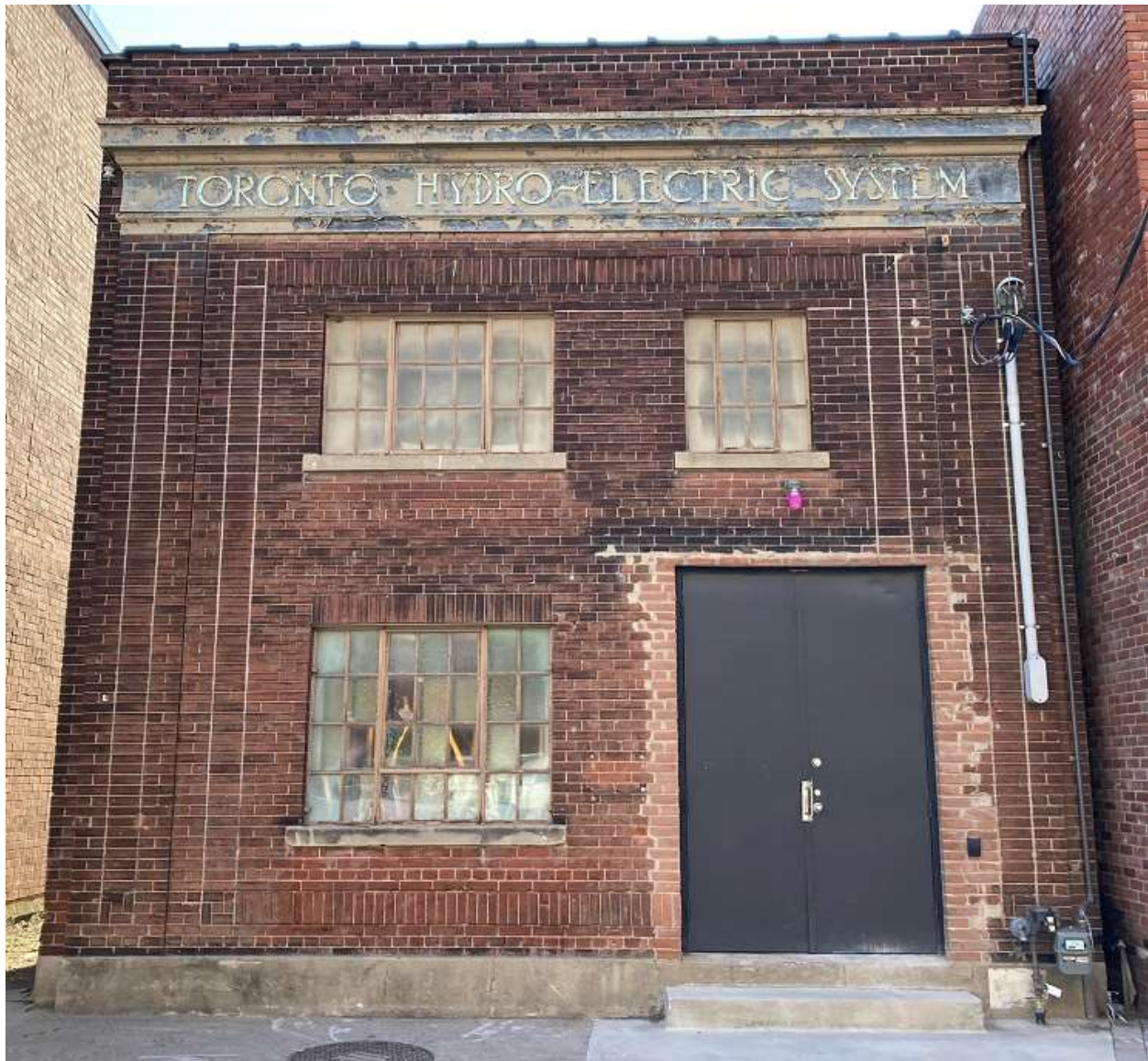
18 Portland Street. Principal (east) elevation. Heritage Planning, 2022.
