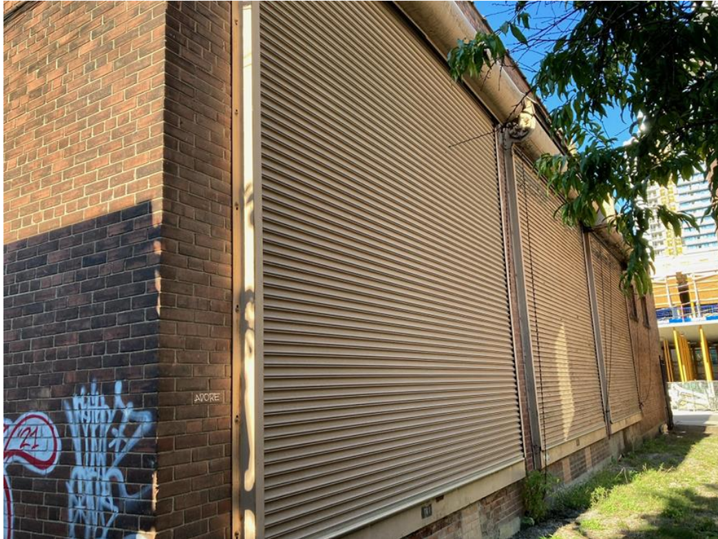
Side (south) elevation of 18 Portland Street
