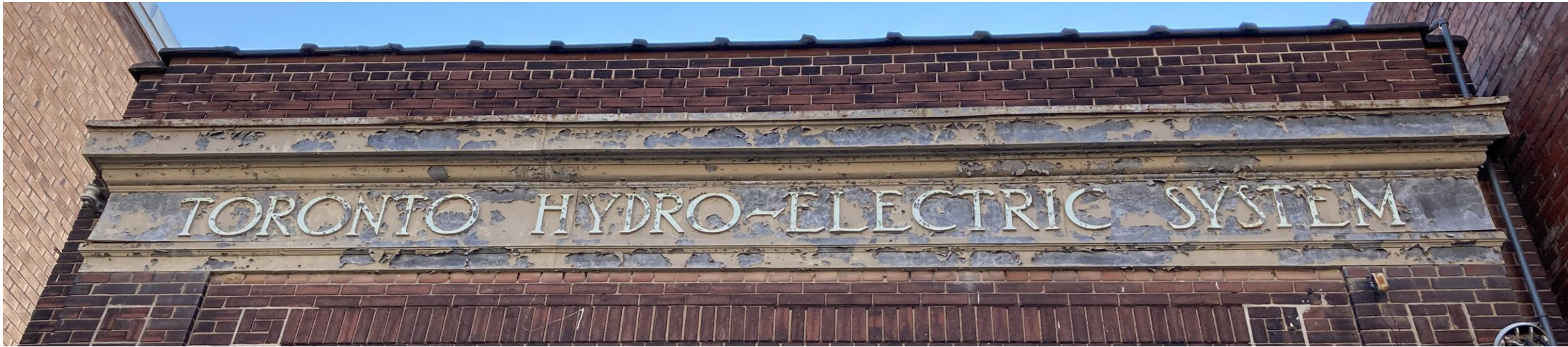
Metal entablature and “TORONTO HYDRO-ELECTRIC SYSTEM” sign band upon the principal (east) elevation of the Portland substation at 18 Portland Street
