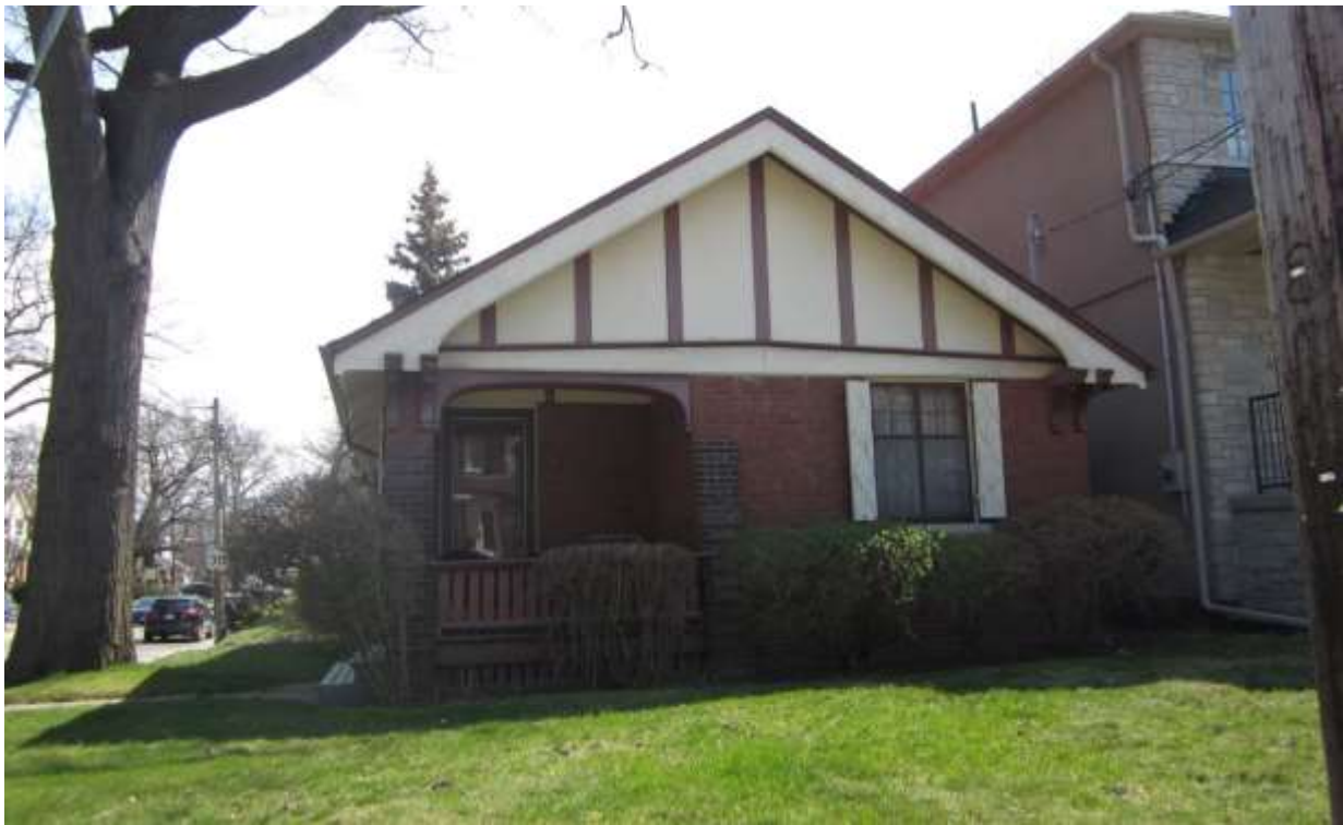
Image 12. Current image of the north elevation
