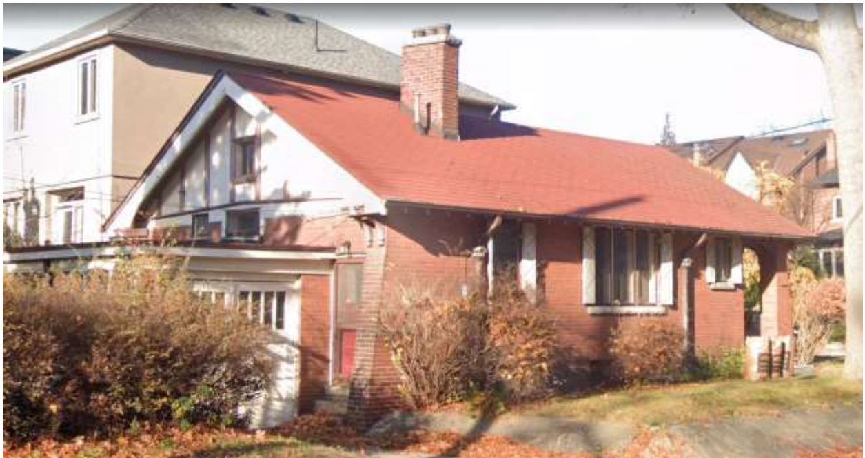
Image 15. Current image looking northwest
