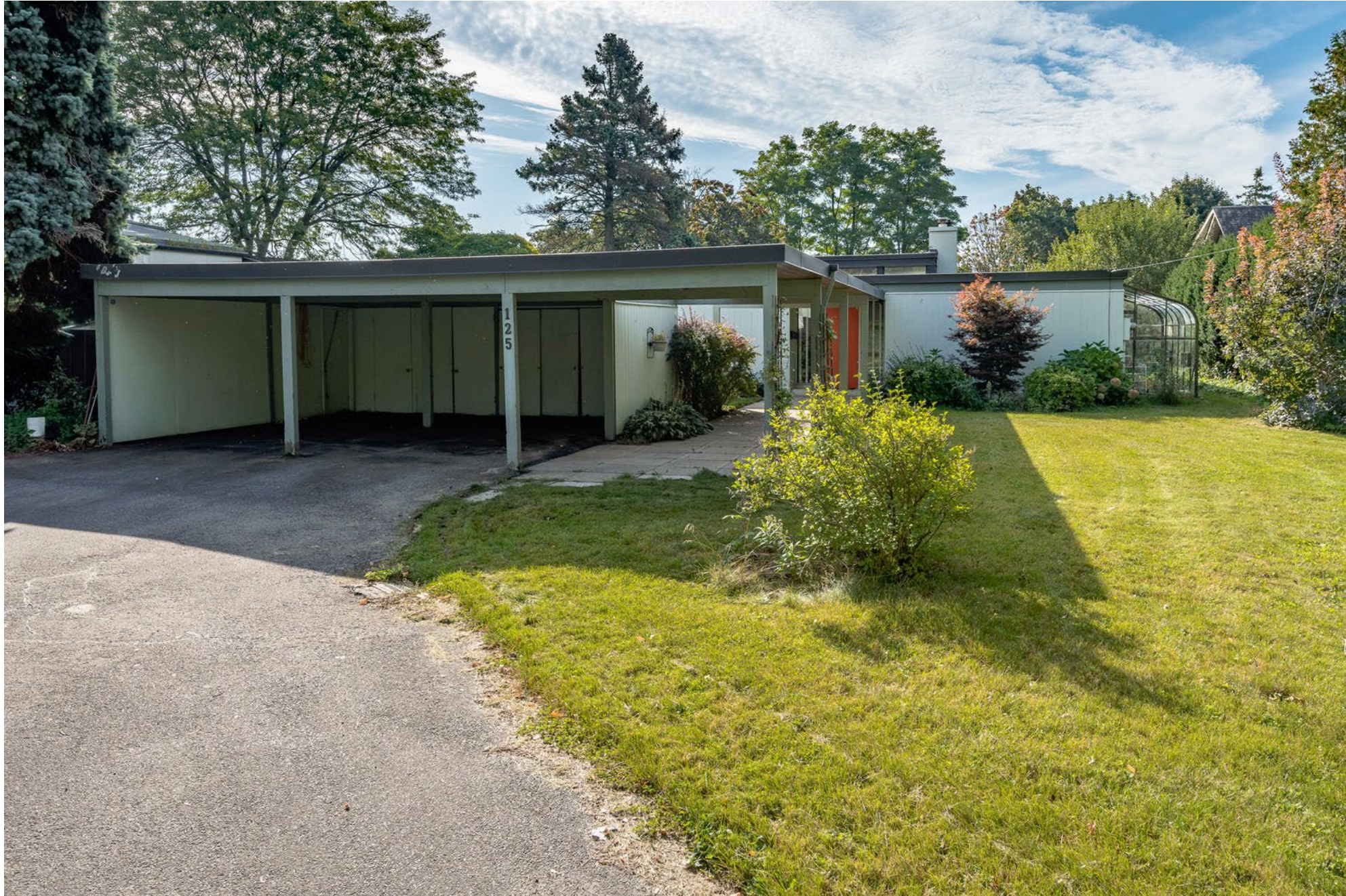
Front (north) elevation photo
