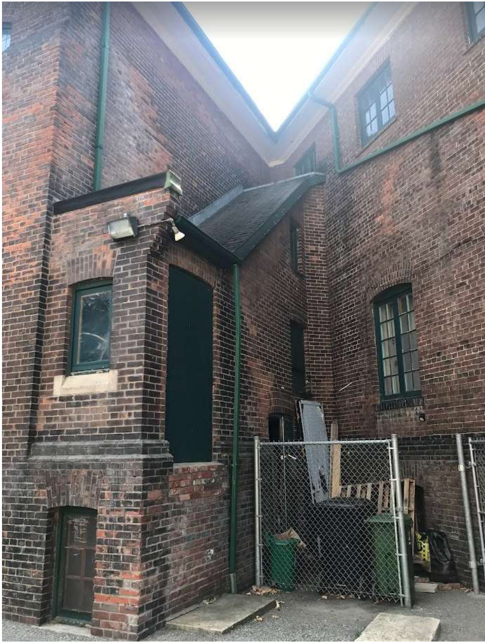
Image 21. Detail of the rear (east) elevation, showing the seamless integration of the 1914 Sunday School wing with the 1907 building. (Heritage Planning, 2022)
