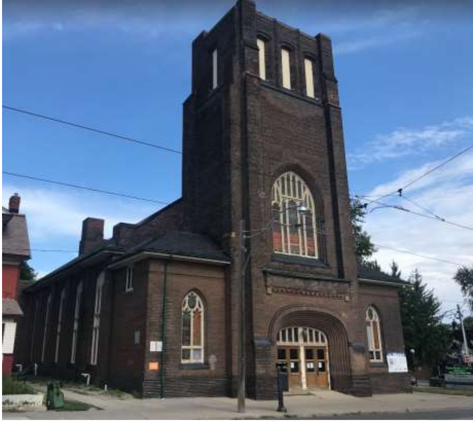
Image 16. The principal (west) and north elevations (Heritage Planning, 2022)
