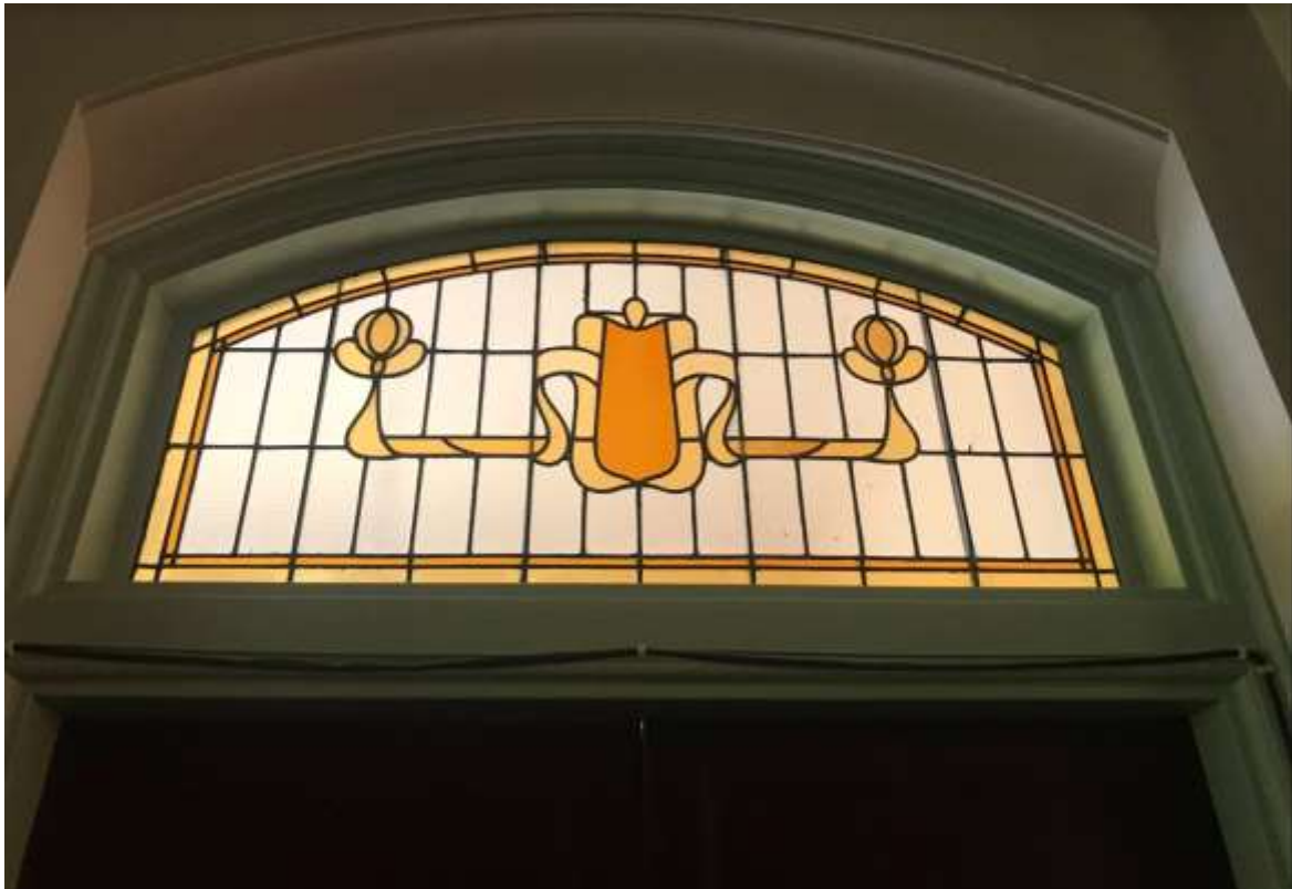
Image 26. Detail of transom and stained glass between the narthex and nave (Heritage Planning, 2022)
