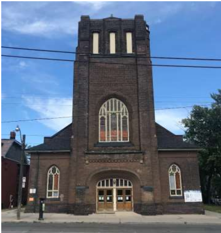
Image 13. Principal (west) elevation of the church with its centred tower and flanking transepts (Heritage Planning, 2022)
