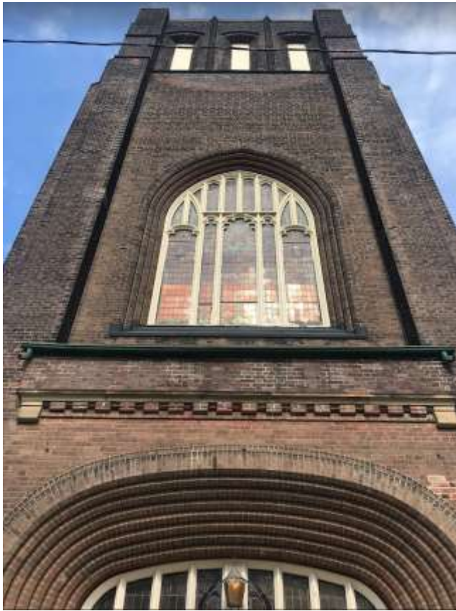
Image 14. Detail of the tower on the principal (west) elevation, showing the Neo-Gothic openings (Heritage Planning, 2022)
