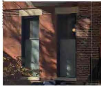
rectangular opening precast & lintel contrast
