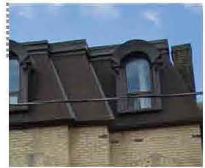
mansard roof dormer window detail
