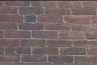
EXISTING REFURBISHED BRICK
