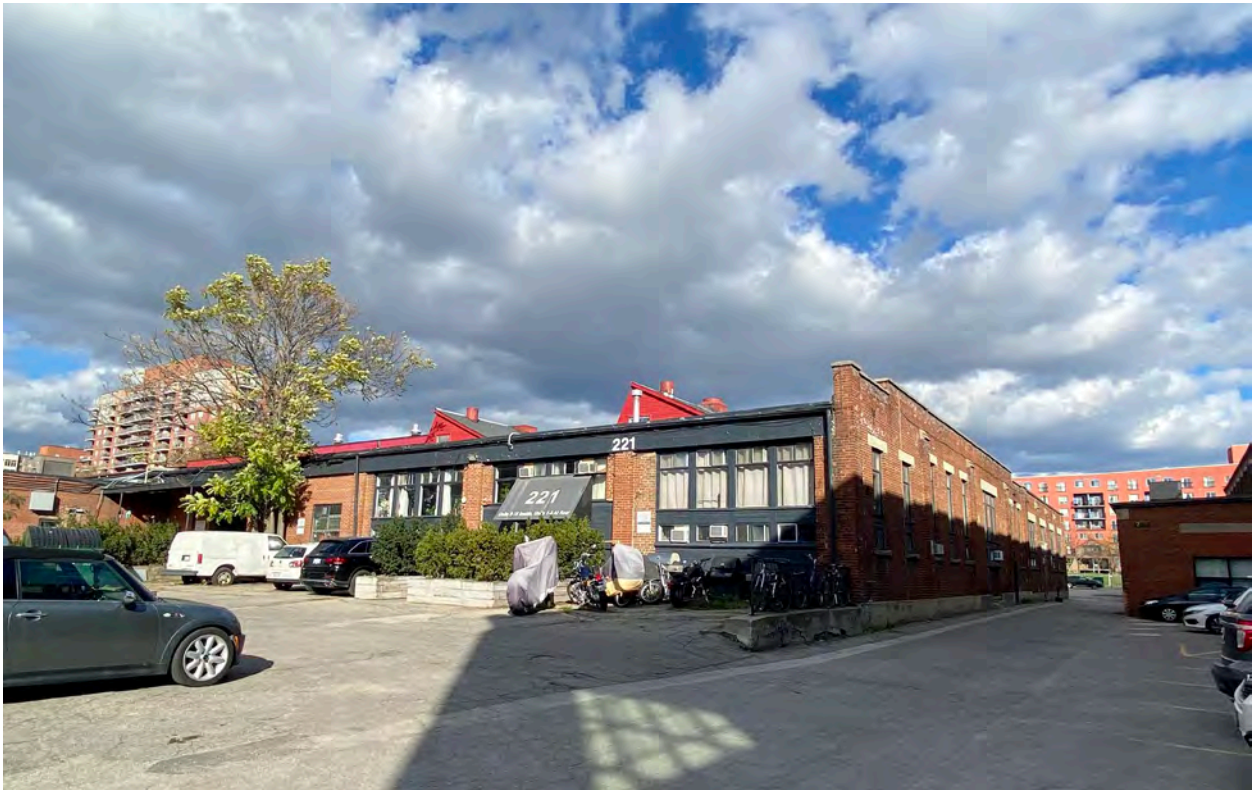
Figure 27: Northeastward view of the subject property's southwestern portion (dating to c.1914-1918). (Heritage Planning, 2021.)
