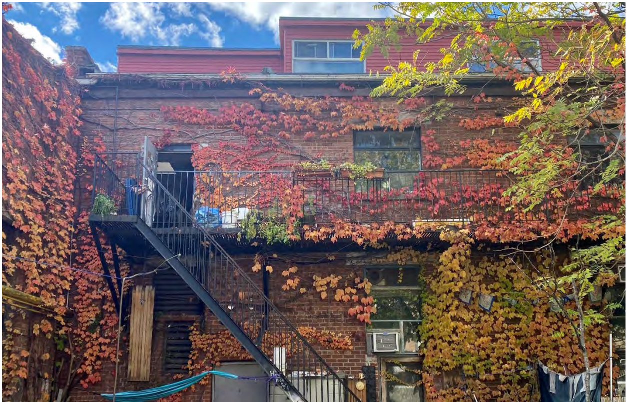
Figure 35: A portion of the subject property's east elevation, dating to c.1924-1939. (Heritage Planning, 2021.)
