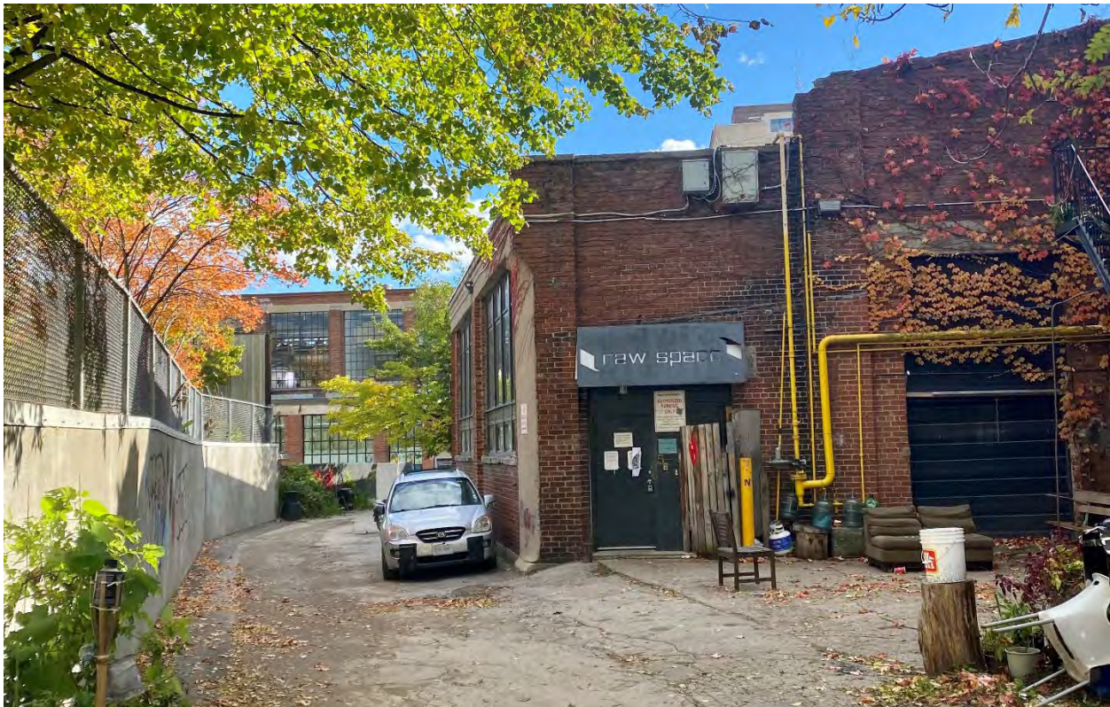
Figure 34: Southward view of a portion of the subject property's east elevation, dating to c.1924-1939. (Heritage Planning, 2021.)
