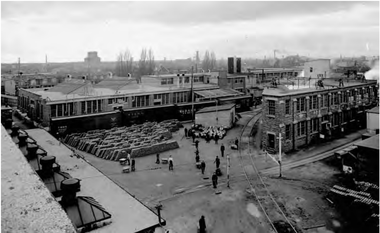
Figure 17: "Section of the Canadian Fairbanks-Morse Co. Ltd. manufacturing department, Toronto, Ont.," believed to date to c.1914-1918. In the background at left, the earliest portion of the extant property at 221 Sterling Road (the southwest portion) is visible in this northwestward view from the adjacent building at 213 Sterling Road.
