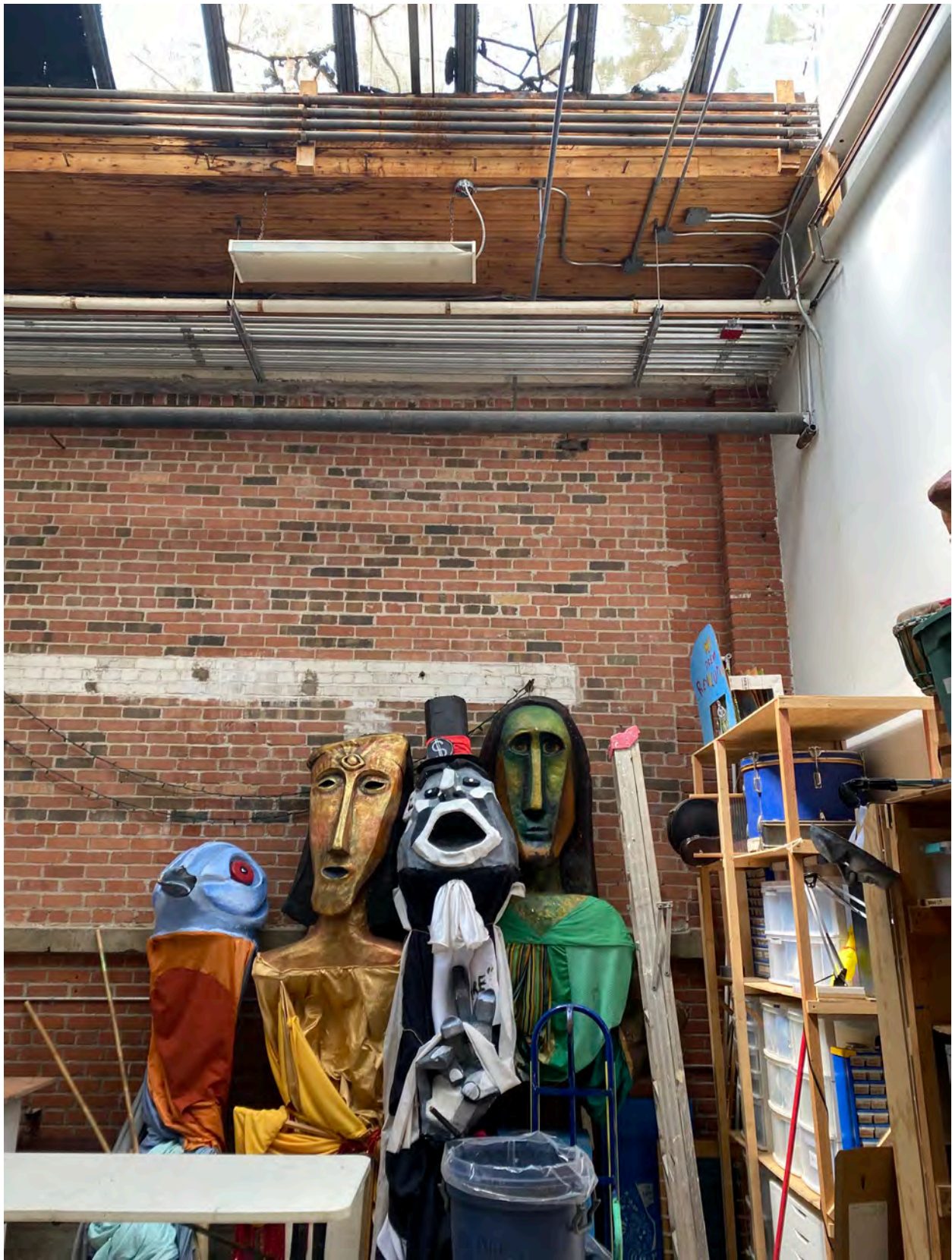
Figure 48: Interior of a unit within the subject property's southern portion, showing high ceiling and skylight; currently used by a theatre company. (Heritage Planning, 2021.)
