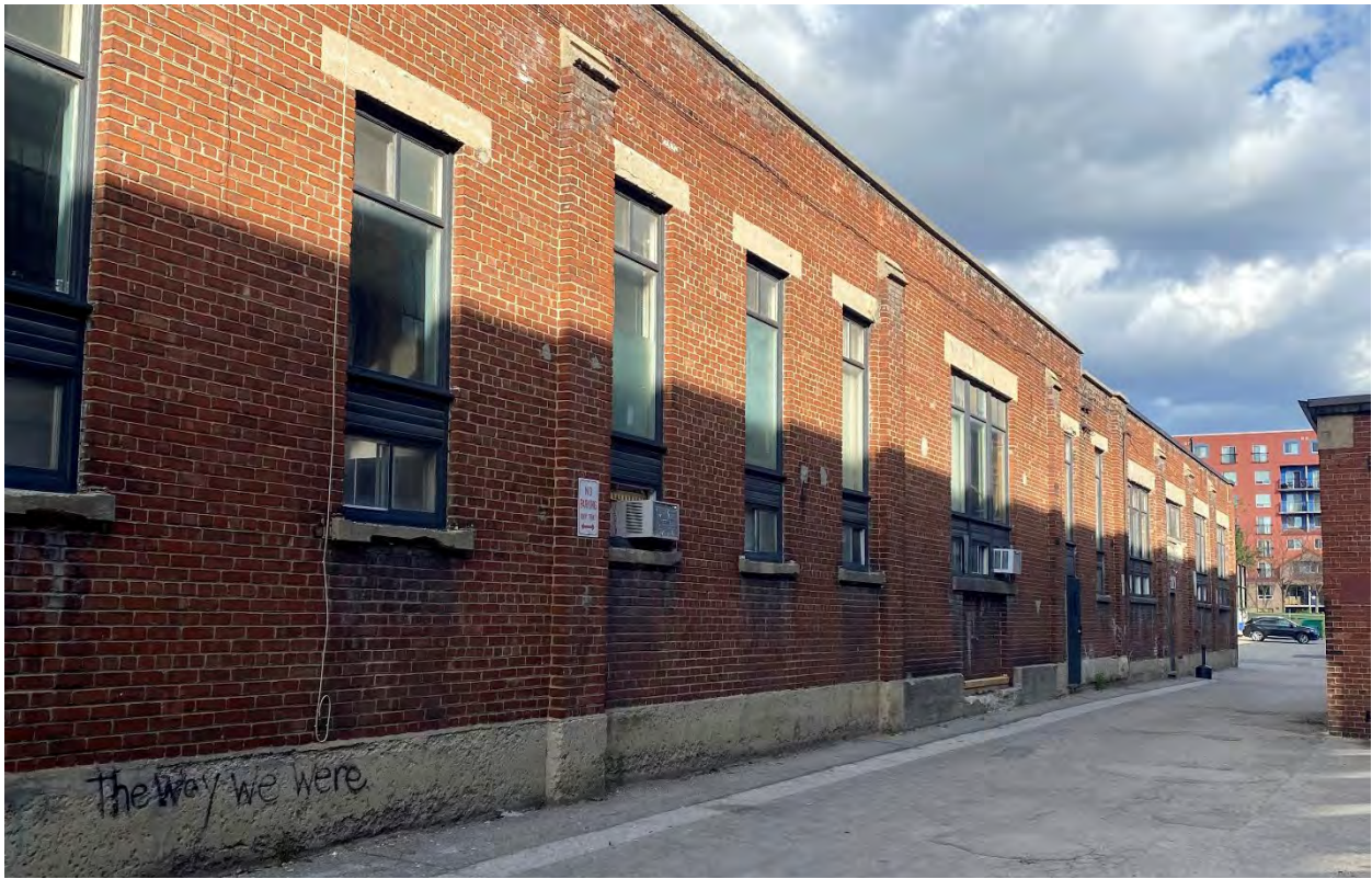
Figure 30: Northeastward view of the subject property's south elevation (dating to c.1914-1918). (Heritage Planning, 2021.)
