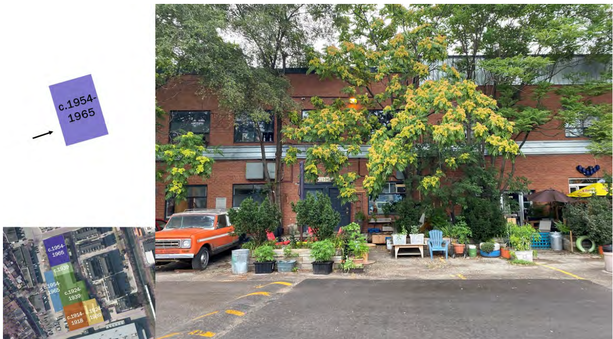
Figure 26: View of the northern c.1954-1965 portion of the building (with arrow indicating direction of view). (Heritage Planning, 2021.)
