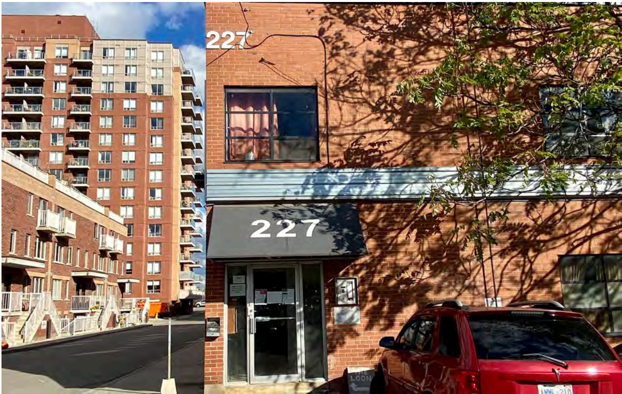
Figure 41: West elevation of the subject property's northern portion (dating to c.1954-1965), including the main entry to this part of the building. (Heritage Planning, 2021.)
