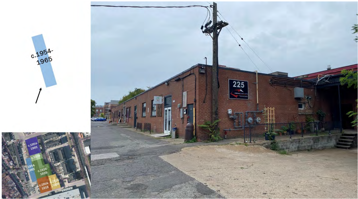
Figure 25: View of the western c.1954-1965 portion of the building (with arrow indicating direction of view). (Heritage Planning, 2021.)
