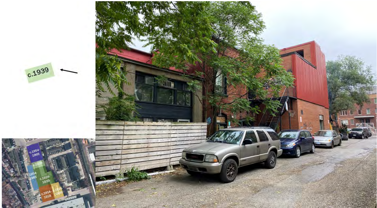
Figure 24: View of the central-northern c.1939 portion of the building (with arrow indicating direction of view). (Heritage Planning, 2021.)
