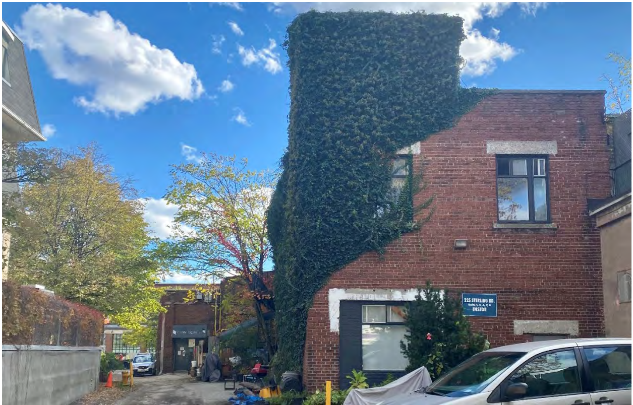
Figure 36: Southward view of a portion of the subject property's east elevation, dating to c.1924-1939. (Heritage Planning, 2021.)
