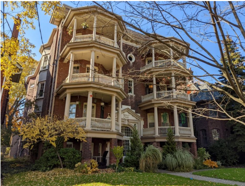
22. Current photograph looking west, showing the south and east elevations of the building at 68 Kendal Avenue (Heritage Planning, 2021).
