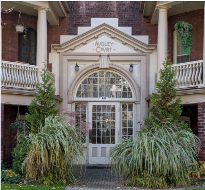
24. Current photograph looking west, showing a detail of the front entrance of 68 Kendal Avenue (Heritage Planning, 2021).
