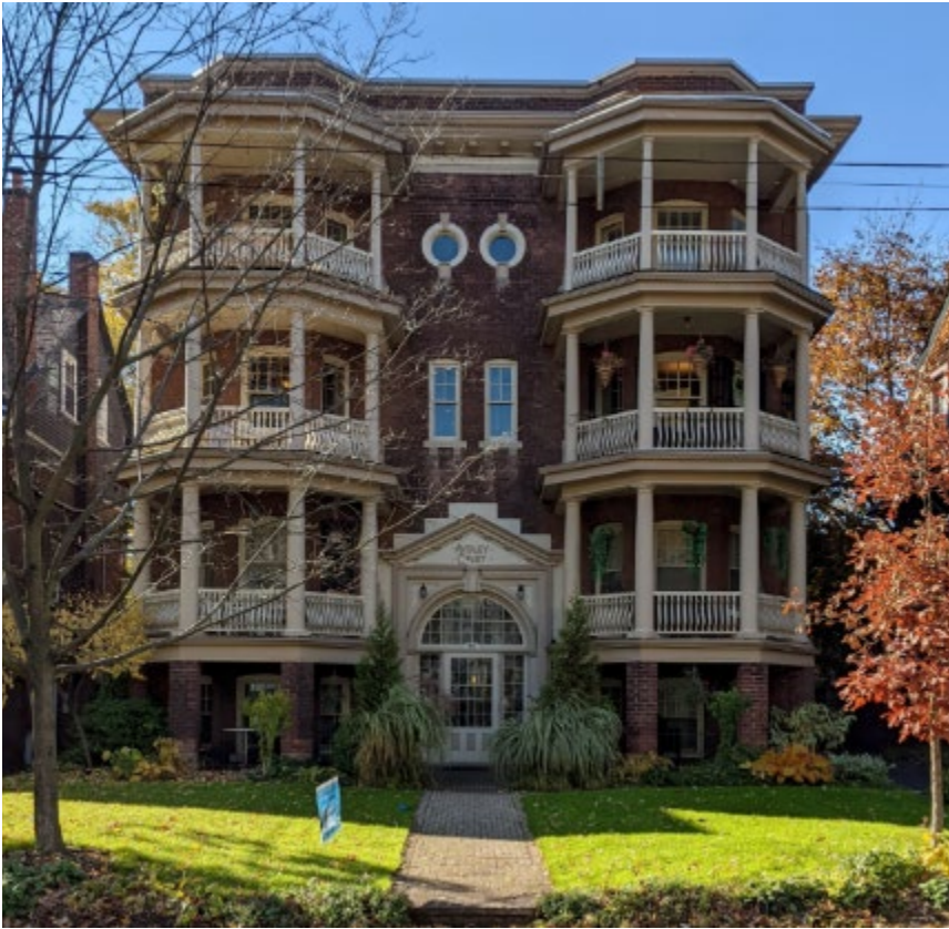
21. Current photograph looking west, showing the east elevation of the building at 68 Kendal Avenue (Heritage Planning, 2021).
