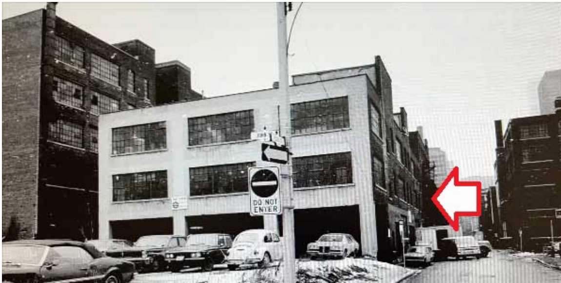
Figure 17. Archival Photograph of 14 Duncan Street in 1973, showing contextual views on Pearl Street, looking east toward Duncan Street (City of Toronto Archives, Fonds 2043, File 202)
