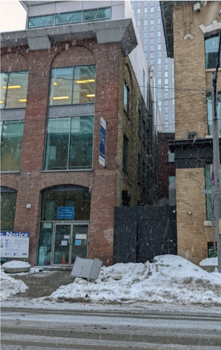
Figure 26. Detail of the side (north) elevation of 14 Duncan Street (Heritage Planning, 2022)
