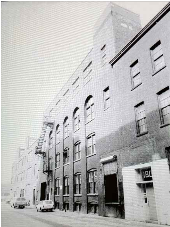
Figure 14. Archival photograph of 14 Duncan Street in 1973, showing the extended south elevation on Pearl Street (below) (City of Toronto Archives, Fonds 2043, Files 79 and 202)
