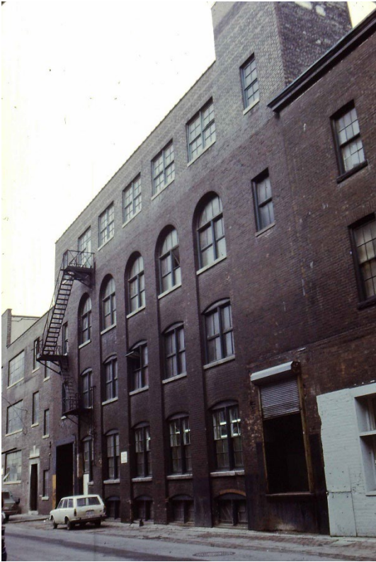
Figure 18. Archival Photographs of 14 Duncan Street in 1973, showing the south elevation on Pearl Street with the 1906 wing and its fourth-floor addition before the alterations to the building (Toronto Historical Board)
