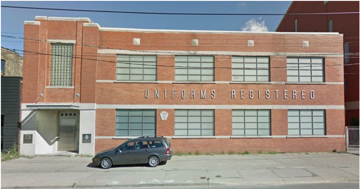
Figure 19: Primary elevation of the subject property, August 2011 (Google Street View).
