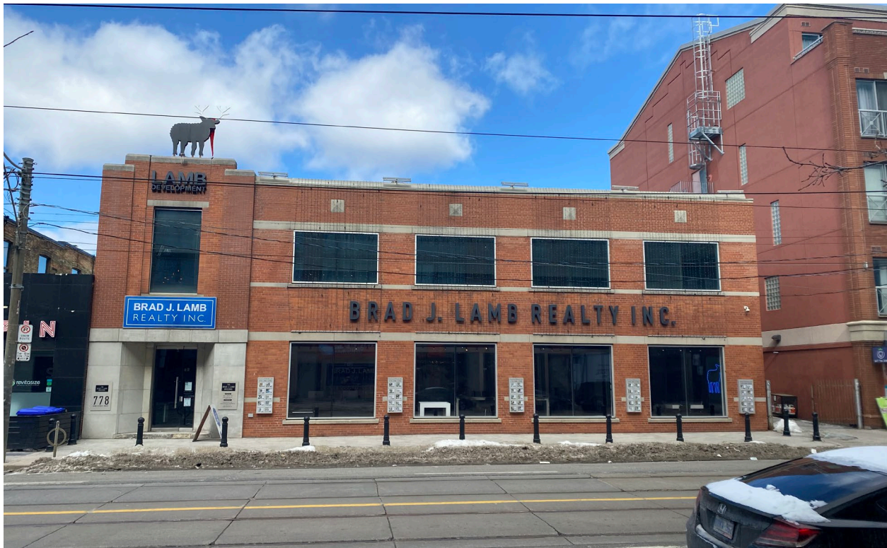
Figure 23: Primary (south) elevation of 778 King Street West (Heritage Planning, 2022).
