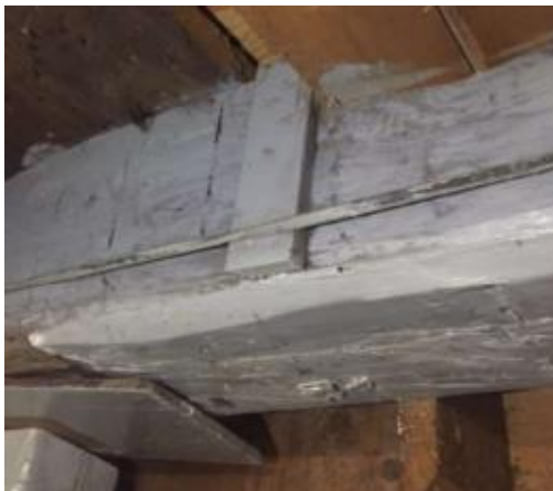
14, 15 and 16. Photos showing the massive timber support beams in the unfinished basement with their hand-hewn markings. (ERA, 2019)
