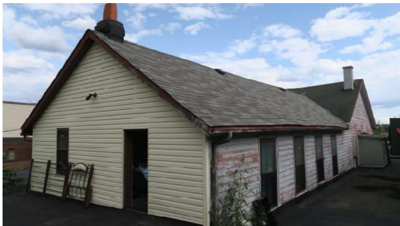
17 and 18. Photos showing the exterior sheathing of the original building including lath and plaster protected by tongue-and-groove wooden siding. At right, the north elevation of the tail is currently over-clad with vinyl siding. (ERA, 2019)
