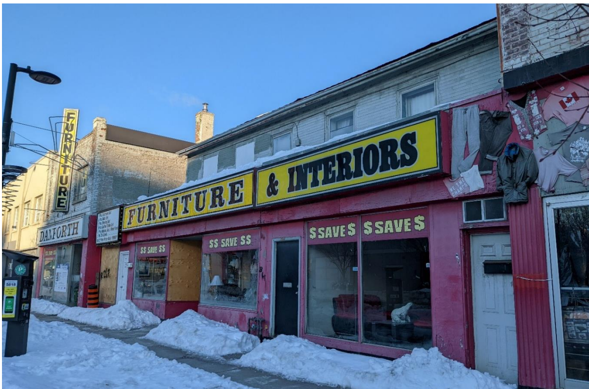
11. Oblique view of the principal (south) elevation at 2726 Danforth, looking northwest. (Heritage Planning, 2022).
