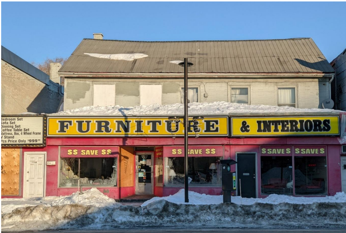
10. Principal (south) elevation of 2726 Danforth Avenue with its early 20th century projecting storefront addition at street level. (Heritage Planning, 2022)
