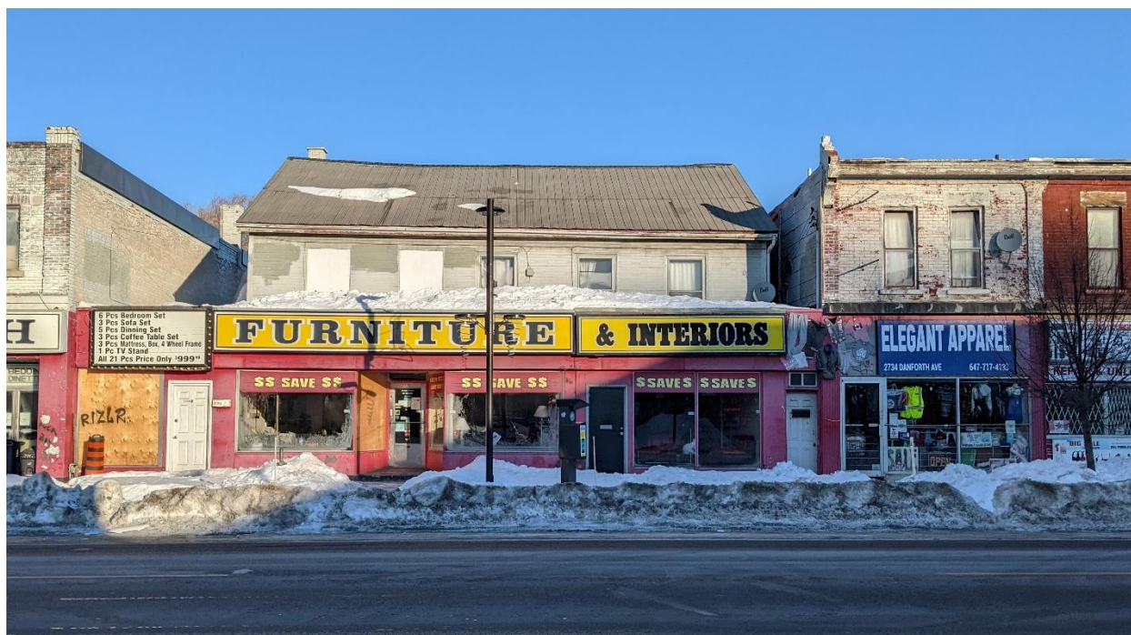
South elevation of 2726 Danforth Avenue at centre and 2734 Danforth Avenue adjacent at right. (Heritage Planning, 2022)
