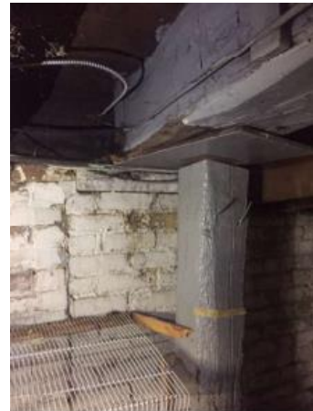
14, 15 and 16. Photos showing the massive timber support beams in the unfinished basement with their hand-hewn markings. (ERA, 2019)
