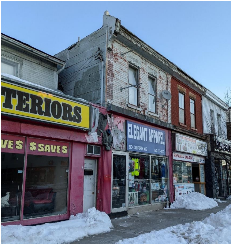
21. Current photo of 2734 Danforth Avenue showing the wooden cornice and decorative corner bracket. Also visible are the two adjacent properties at 2736 and 2740, which were built together with the subject property in c.1886 (Heritage Planning, 2022)
