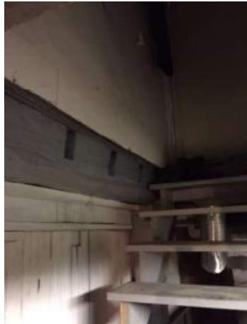
14, 15 and 16. Photos showing the massive timber support beams in the unfinished basement with their hand-hewn markings. (ERA, 2019)
