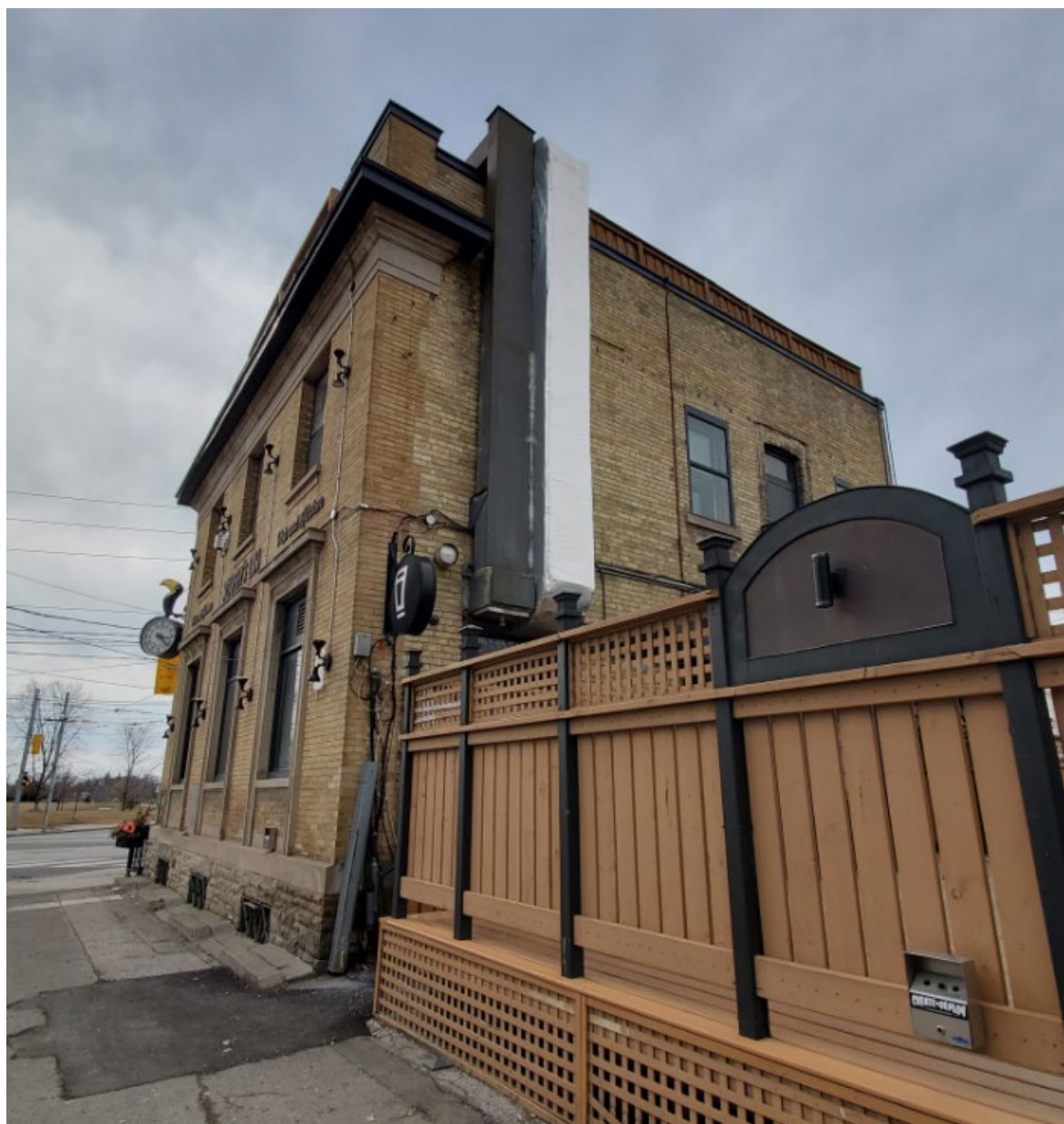
Figure 15. Detail of the corner quoining in the rear (north) elevation of 1702 Queen Street East (Heritage Planning, 2022)
