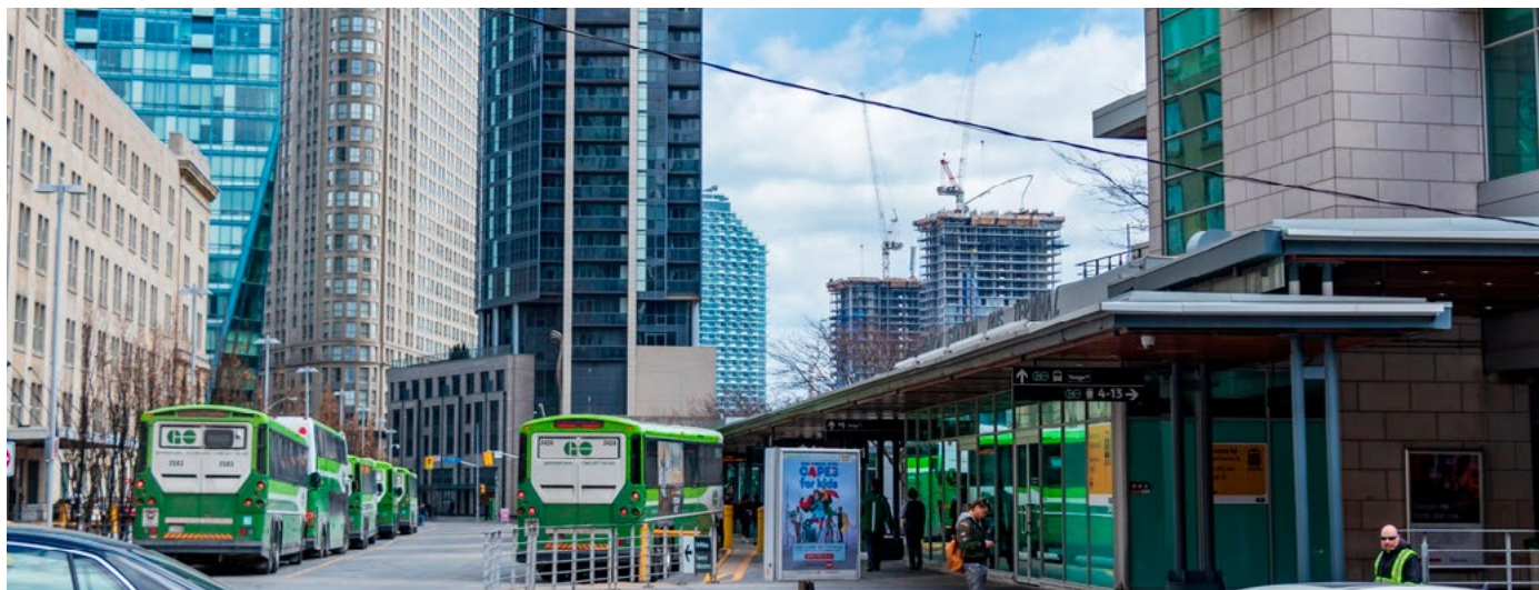
Figure 8: Union Station Bus Terminal, Toronto (Photo Credits: JL Images, Shutterstock)
