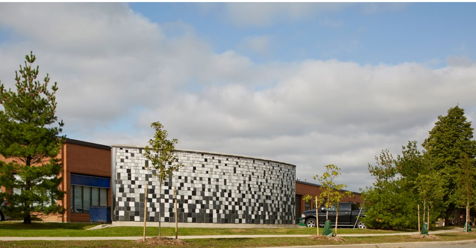
Figure 9: Emergency Exit Building along the Toronto-York Spadina Subway Extension (Photo Credit: Ben Rahn/A-Frame Studio)
