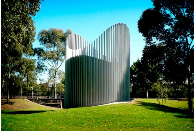
Figure 4: Transgrid Ventilation Shaft, Queensland (Photo Credit: Choi Ropiha Figuera)
