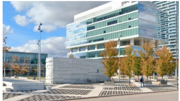
Figure 13: EEB and vent shaft, Vaughan Metropolitan Centre
