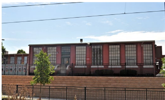
Figure 19: Substation after a commissioned artist's treatment allows it to blend it more seamlessly into the surrounding context (Photo Credit: Leigh Brinkley, City of Charlotte)
