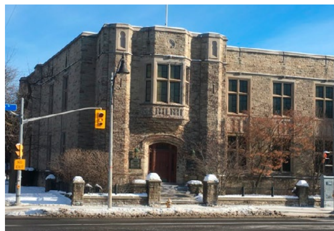
Figure 9: Hydro substation at Yonge and Glengrove (Photo Credit: HikingtheGTA.com)
