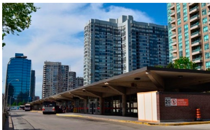
Figure 9: Bus Network configured to provide heavy service to the current subway terminus at Finch Station, Toronto (Photo Credit: TTC, Wiki Commons)
