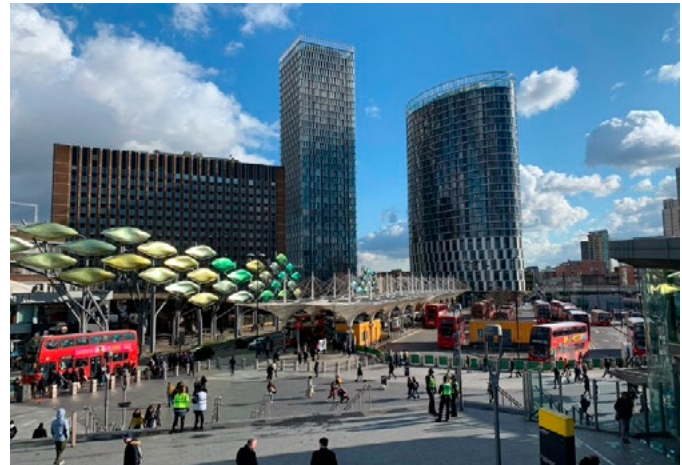
Figure 46: Visual cues to and through the bus terminal promoting ease of transfer and permeability to surrounding uses, London, Stratford, UK (Photo Credit: Marcus Bowman)
