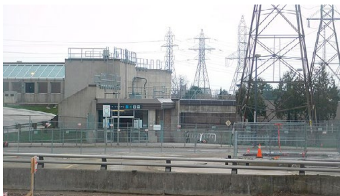
Figure 16: Hydro Corridor condition at Kipling Station (Photo Credit: Wiki Commons)
