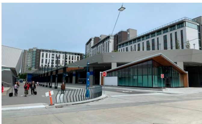
Figure 13: Integrated facility, UBC Exchange (Photo Credit: Marcus Bowman)
