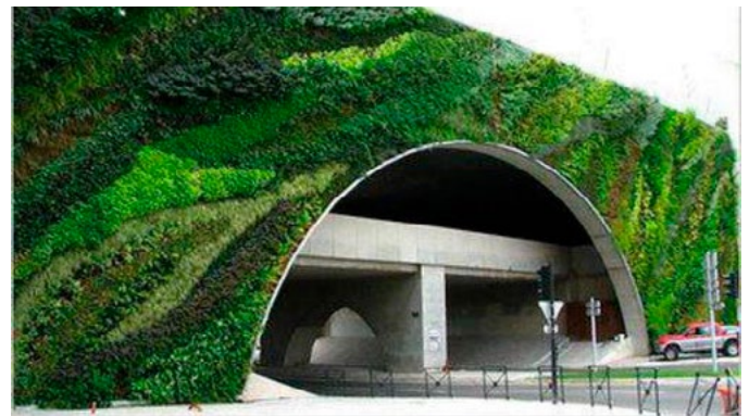
Figure 18: Vertical green walls (Photo Credit: Patrick Blanc)
