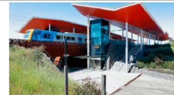
Figure 5: Middle George Station, Mernda Rail Extension 2, Victoria, Australia (Photo Credit: Level Crossing Removal Project)
