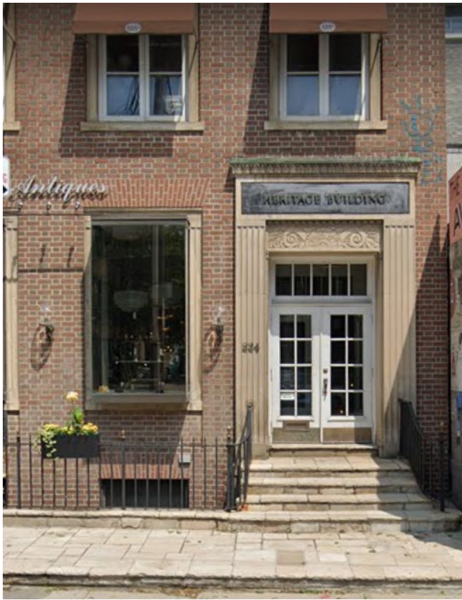
25. 224 Davenport Road: detail of raised main entrance on the principal (south) elevation showing the stone door surround with fluting pilaster and carved inset, decorative window surrounds and metal railing. (Heritage Planning, 2021)
