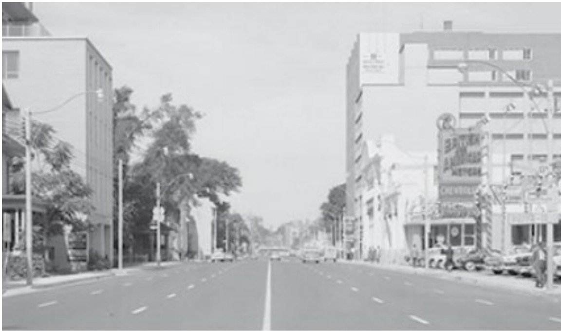
8. 1959 archival photo looking north up Avenue Road from Davenport following Avenue's widening (CTA)
