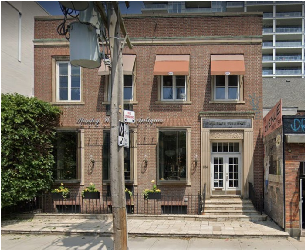
19. 2021 image showing the principal (south) elevation of the former Canada Bread Company head office building at 224 Davenport Road. (Heritage Planning)
