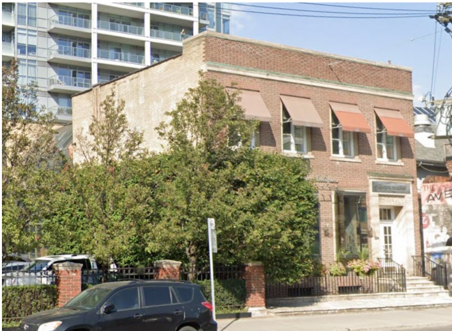
26. Current image of the Canada Bread Building at 224 Davenport Road showing the stone and copper cornice line on the principal (south) elevation and buff brick cladding on the west elevation. (Heritage Planning, 2021)
